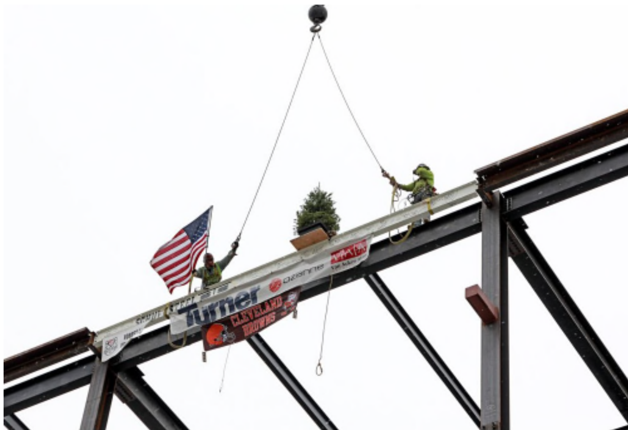
Hilton Cleveland Downtown, Cleveland, Ohio Contract Number: 140177 Photo 155 - Structural Steel Topping Out Date: November 13, 2014
