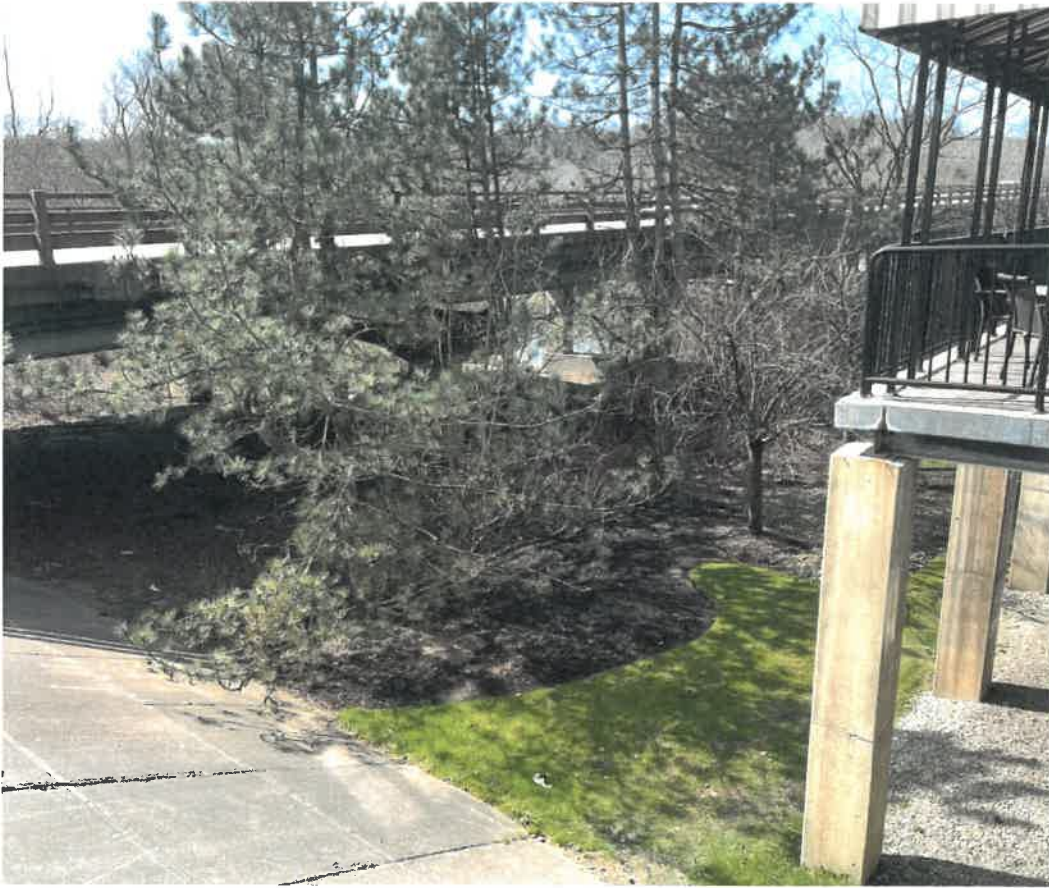
Facing southwest at 10 T
