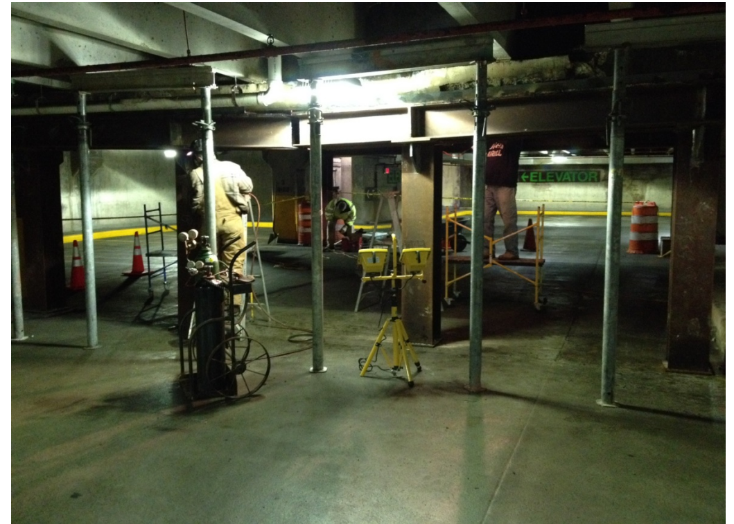
Emergency shoring had to be provided for this girder in Dec. 2014
