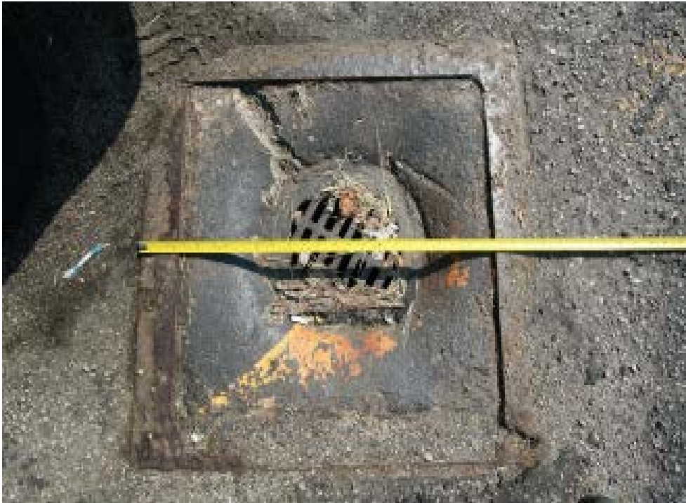
Original roof drain
