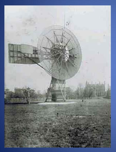
First wind-powered electricity generator, 1888
