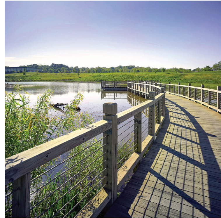
TREATMENT WETLAND WITH BOARDWALK ACCESS
