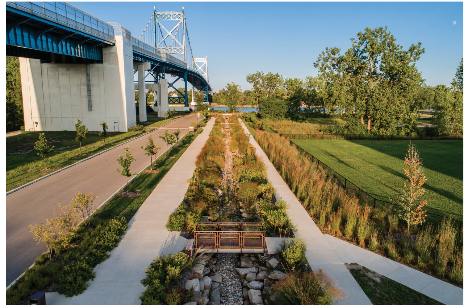
CLEAN RUNOFF FROM BRIDGES AND CREATE AN AMENITY
