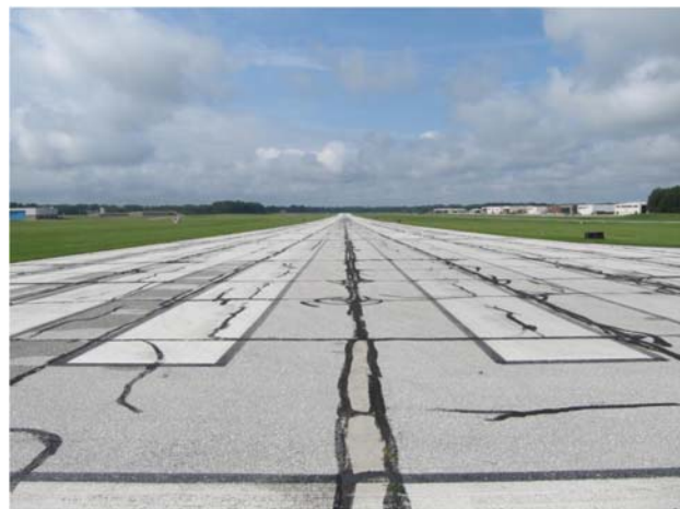
Photo of Current Runway Condition
