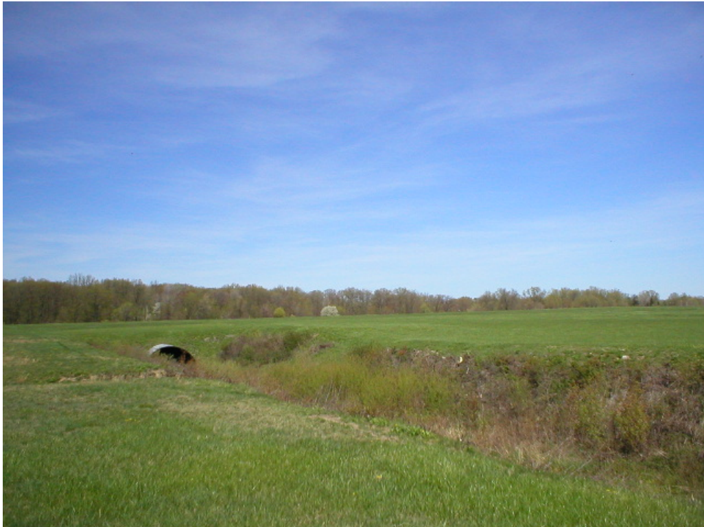
View of culvert, located near Bishop Road, looking northeast
