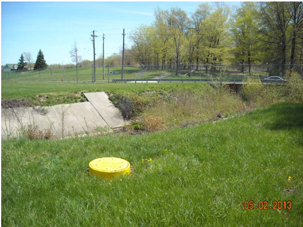
View of storm sewer access near Bishop Road
