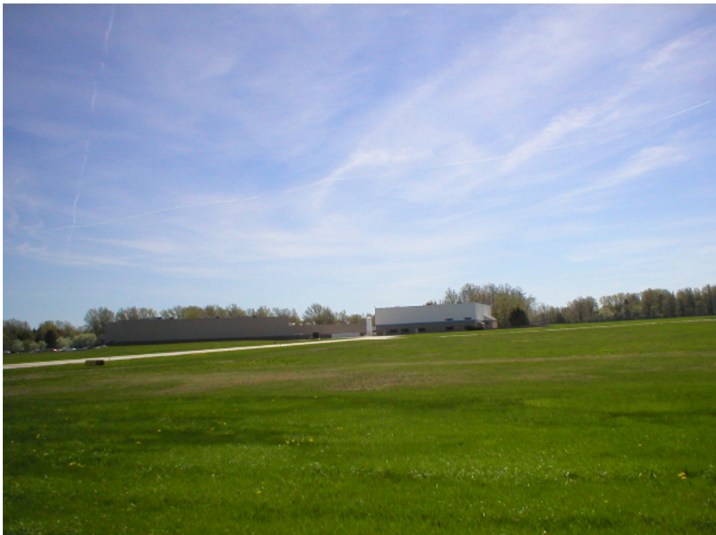
View of taxiway B, looking south
