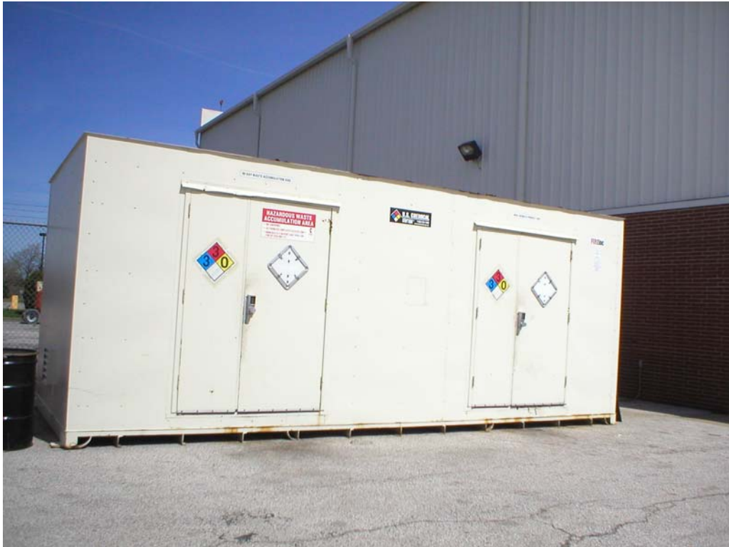
View of hazardous materials storage building, located south of the Corporate Wings hangar
