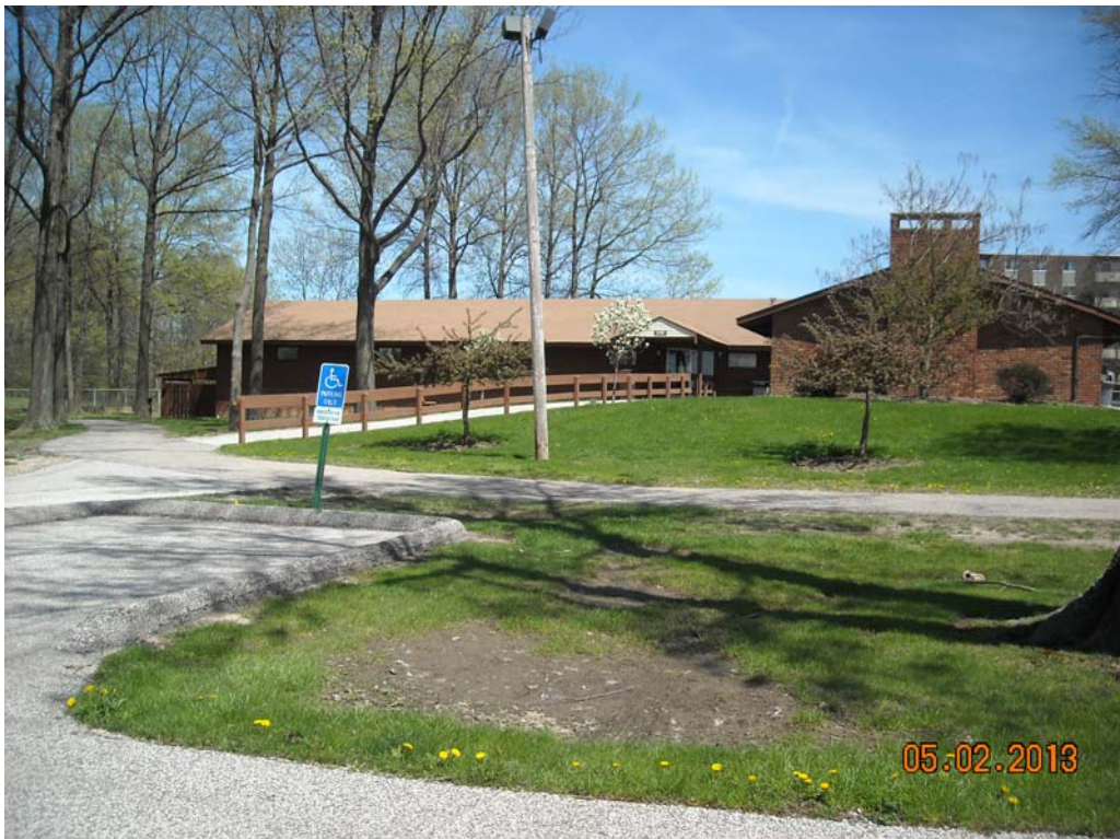
View of Kiwanis building located along the southern property boundary
