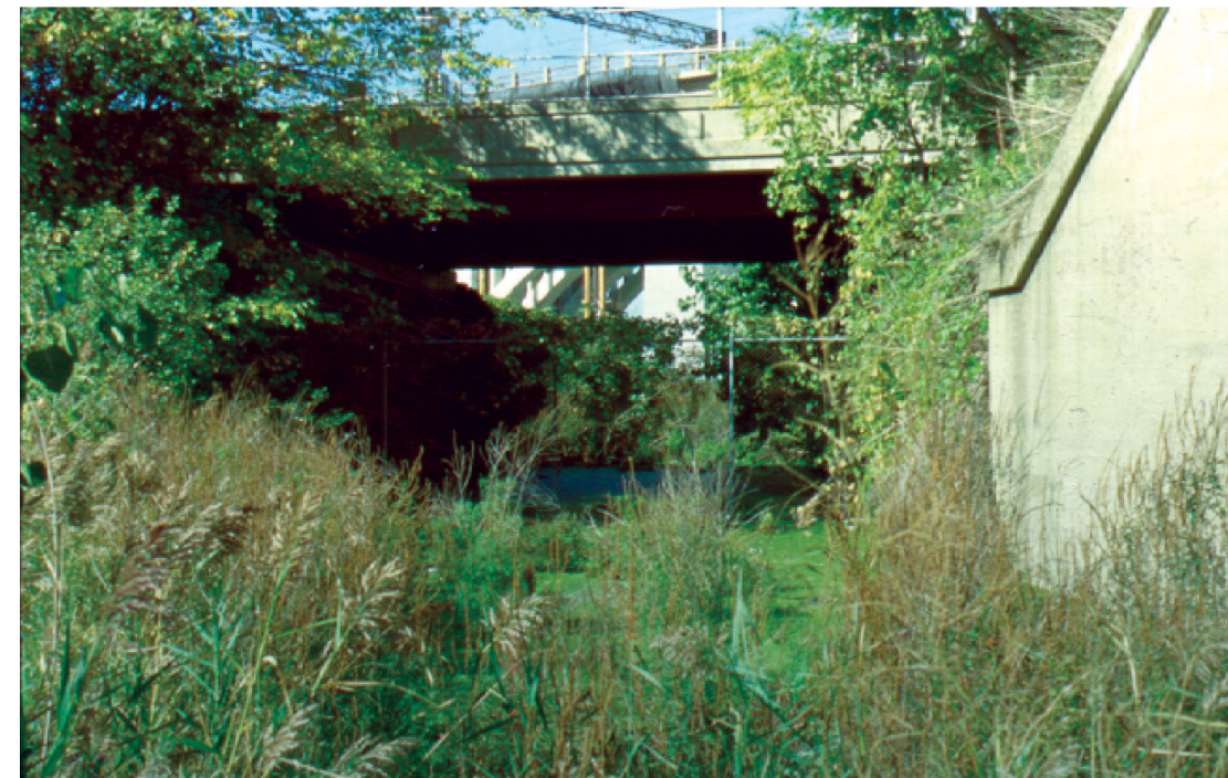
Original bed of Ohio & Erie Canal under Columbus Road at Sherwin-Williams
