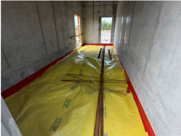
Prep Slab on Grade at Stair Core
