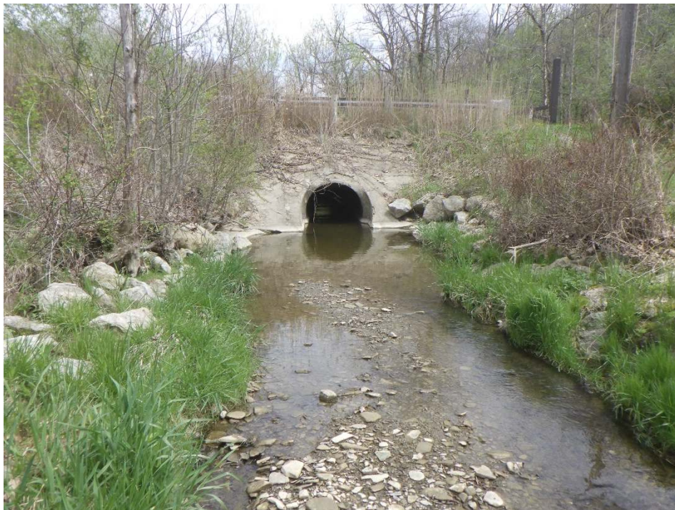
Photograph No. 12 – View of the culvert conveying Stream 2 under a roadway, facing east (EMH&T 5/5/2022).
