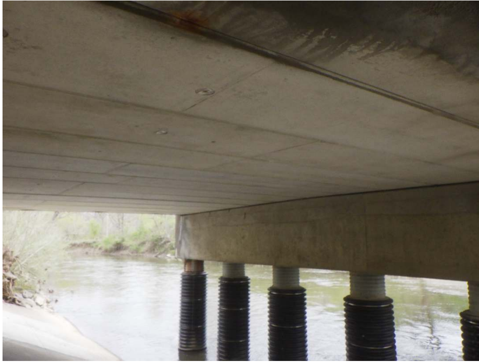
Photograph No. 13 – Upstream view of the Cuyahoga River along the eastern end of the assessment area, facing north (EMH&T 5/5/2022).
