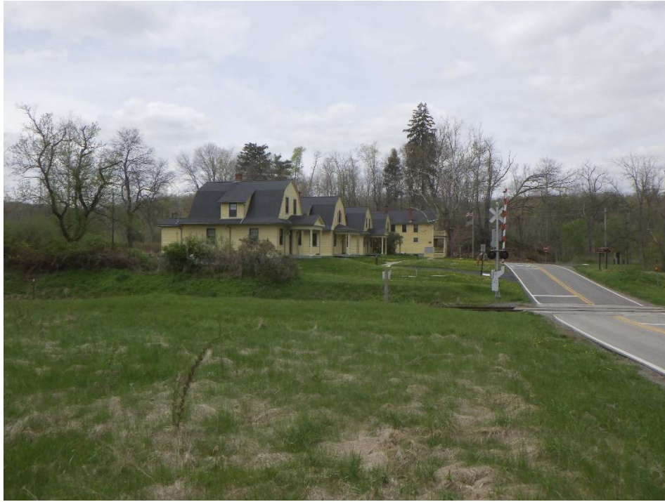
Photograph No. 25 – Overview of the historic park offices within the western part of the assessment area (EMH&T 5/5/2022).
