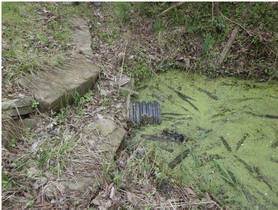
Photograph No. 8 – View of the culvert conveying Stream 1 under Vaughn Road (EMH&T 5/5/2022).
