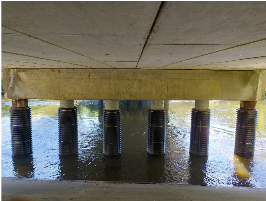
Photo 6 – Facing west - Bent 2 east elevation.
