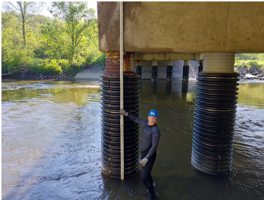
Photo 14 – Clearance level measurement - Bottom of Bent 1 cap at Pile 1.
