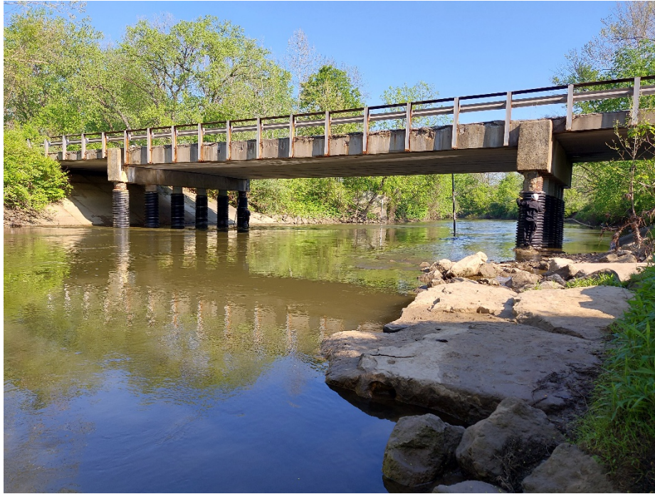
Photo 1 – Facing northwest - South elevation of the bridge.
