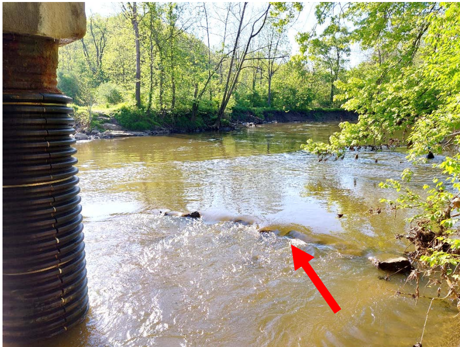
Photo 8 – Submerged rocks creating flow turbulence upstream of Bent 1.
