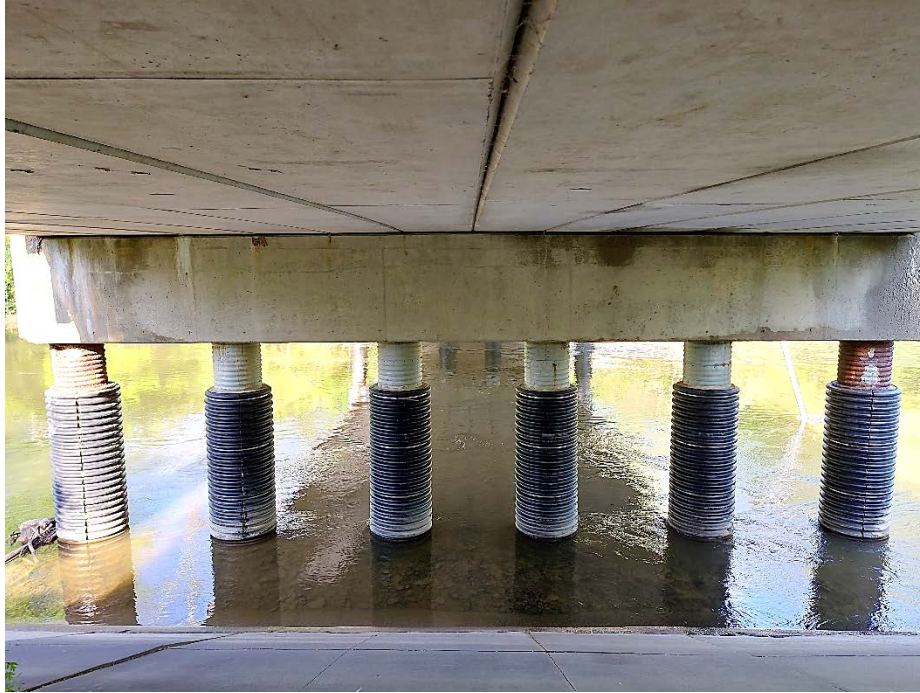
Photo 5 – Facing east – Bent 1 west elevation.
