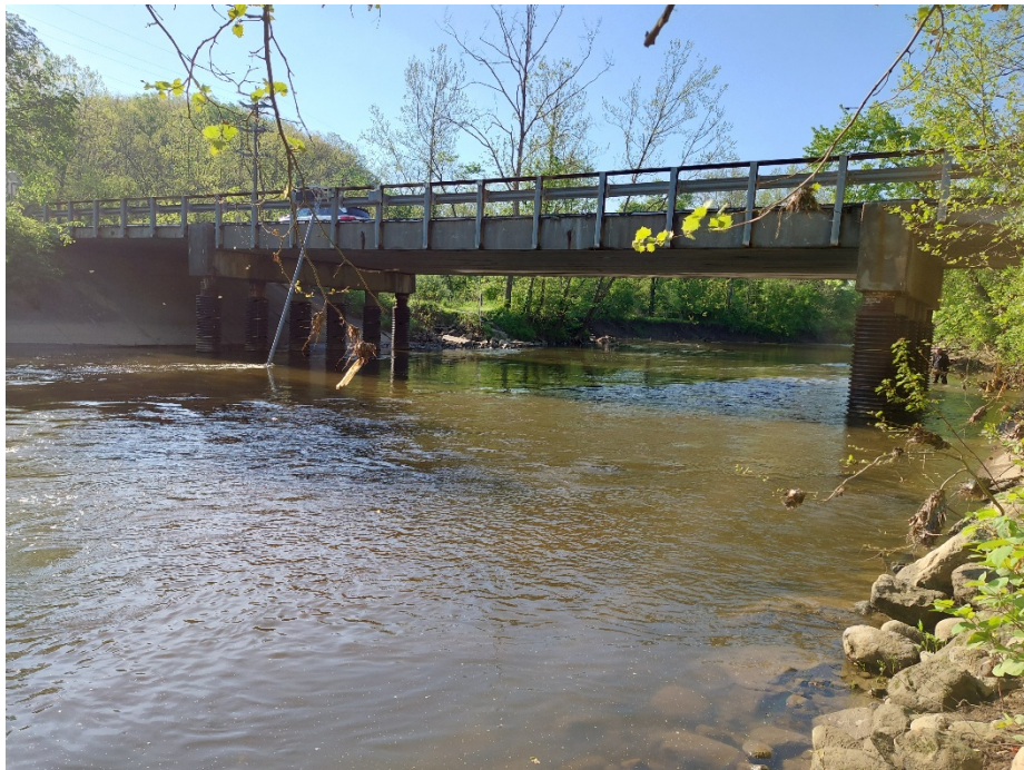
Photo 2 – Facing southeast - North elevation of the bridge.
