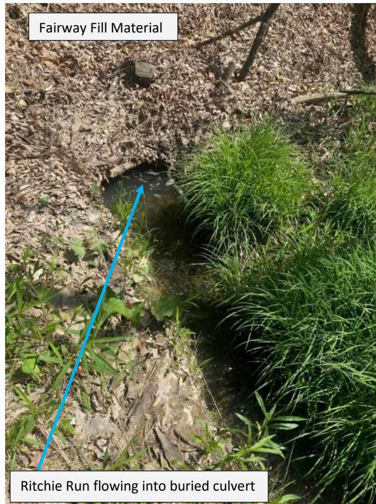
Figure 15: Ritchie Run flowing into buried culvert
