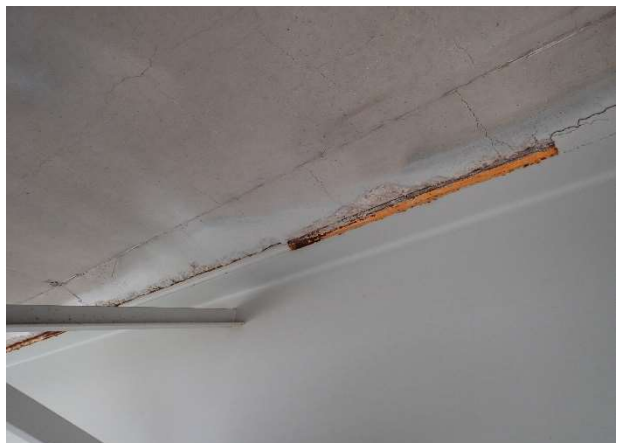
Photograph 132: Span 4 Bay 8 moment plate rusted
