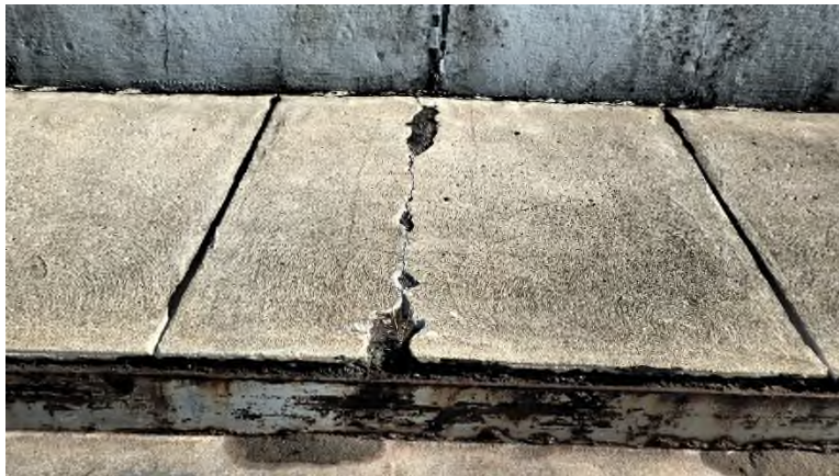
Photo DCK-16: Transverse cracks/minor spalls in right sidewalk
