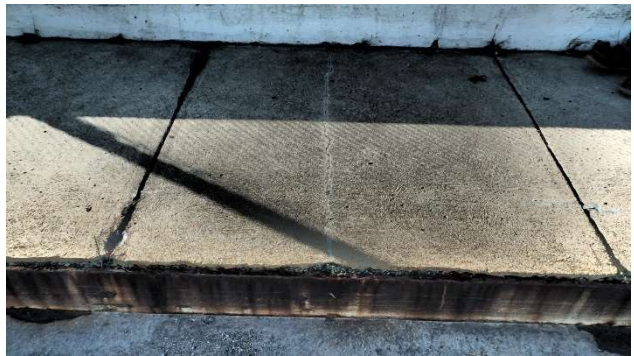
Photograph 350: Span 8 Sidewalk delam and spall 1'x1'
