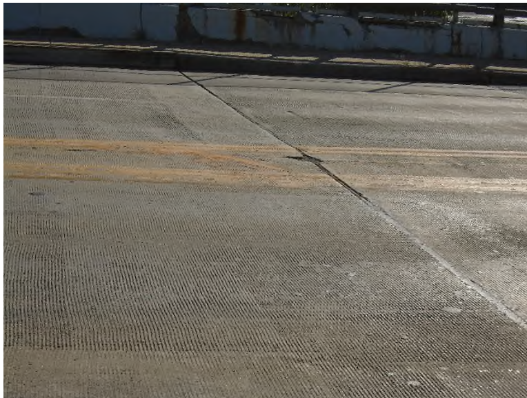
Photo APR-3: Rear Approach (looking east), minor spall in approach slab & concrete pavement (near centerline)
