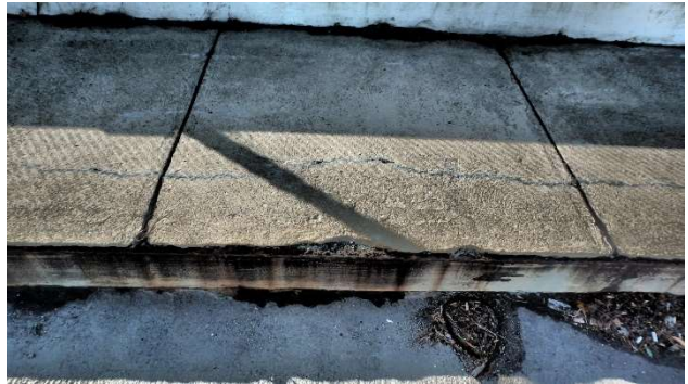
Photograph 278: Span 7 Sidewalk delam and spall 1'x2'
