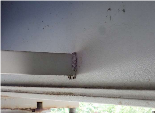
Photograph 99: Span 3 Bad x-frame weld
