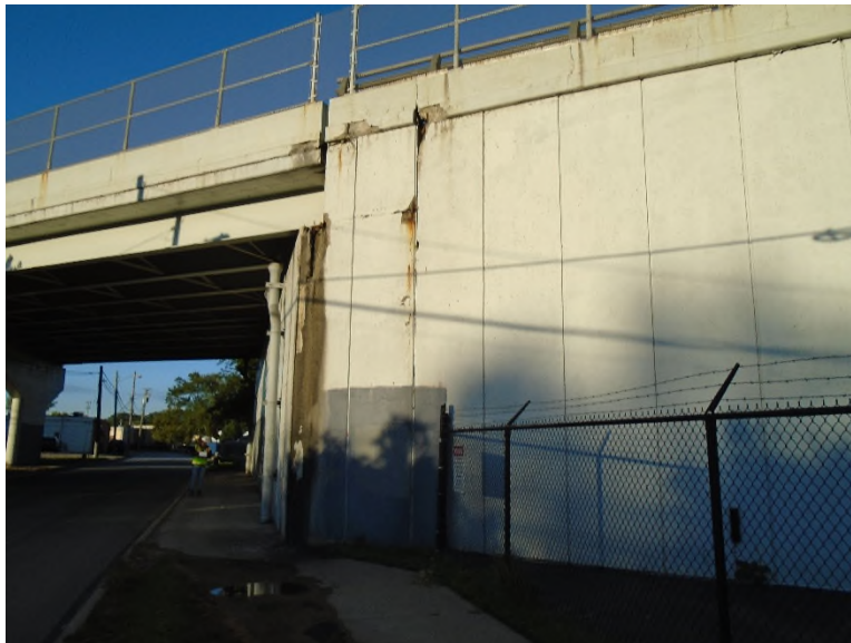
Photo SUB-13: Forward-right wingwall, cracking and minor delaminations/spalling
