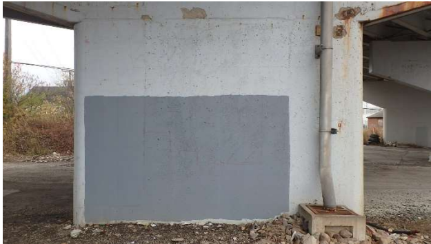
Photograph 247: Span 6 Missing VPF panel @ light pole
