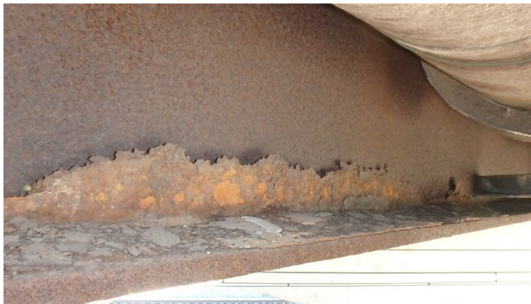
Photo SUP-9: Beam6/Span 8, sheet/pack rust at web and bottom flange in bay 5.
