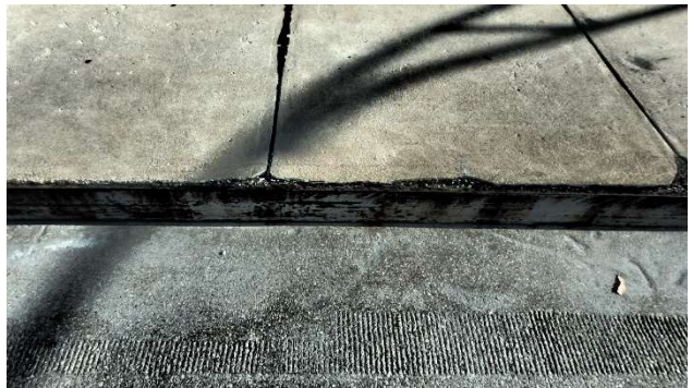
Photograph 266: Span 6 Sidewalk parapet minor cracking and scaling
