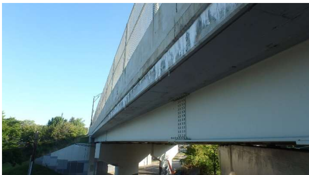
Photograph 351: Span 8 Sidewalk delam and spall 12'x1'
