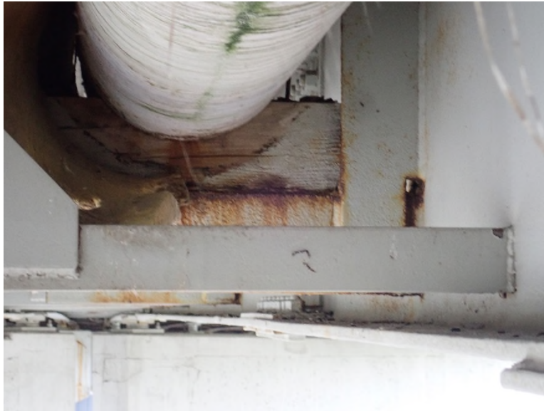
Photo UTL-5: Corroded water-line support angles.
