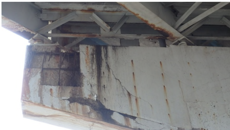
Photo SUB-20: Pier 5L, extensive spalling/deterioration at left end of cap
