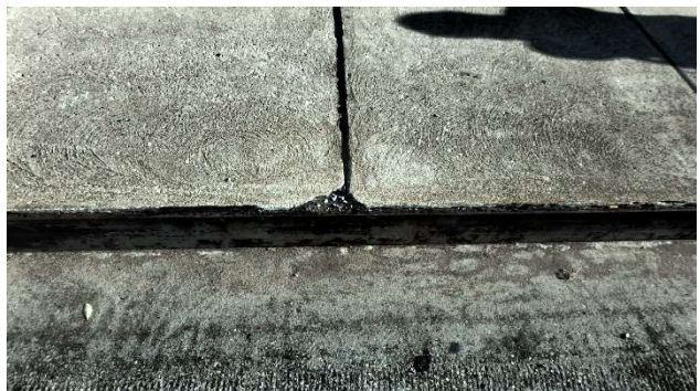
Photograph 358: Span 9 Parapet horizontal and vertical cracking
