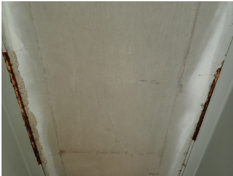
Photo DCK-4: Cracked/spalled haunches along top flange moment plate.
