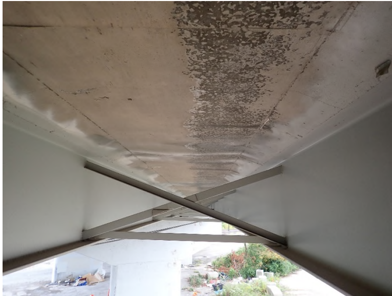
Photo DCK-3: Dark/mottled concrete (~30 wide) in exterior bays (typ. all spans)
