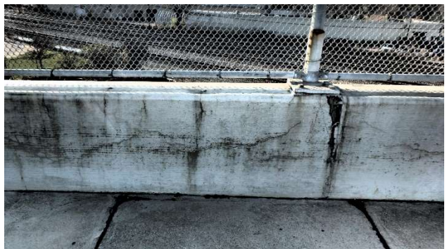
Photograph 112: Span 3 Bay 8 top moment plate rusted S
