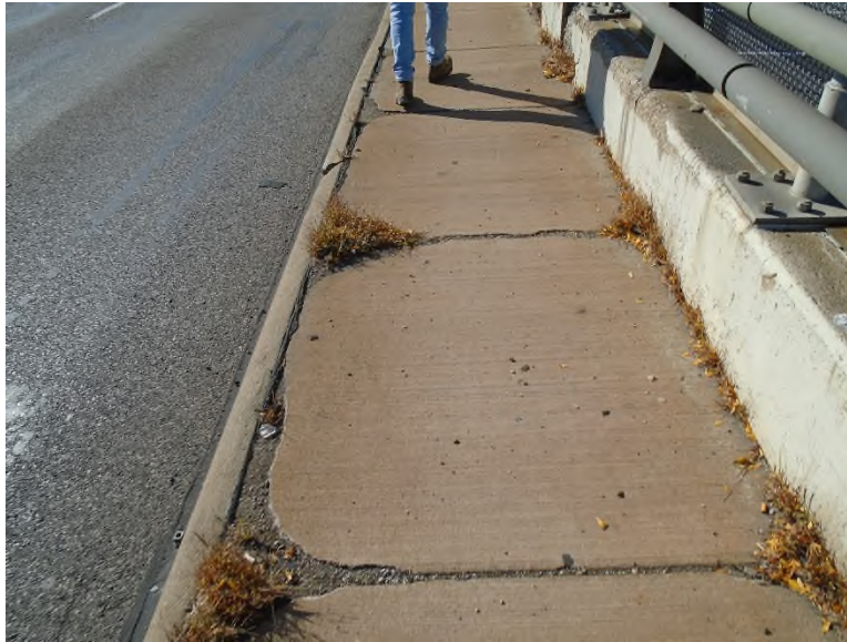
Photo APR-7: Rear-Left Sidewalk, spalled areas and vegetation (typical)
