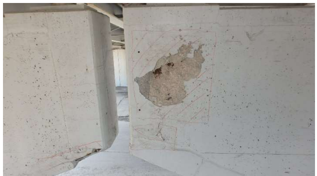
Photograph 94: Span 2 Rusting on web, bm 6, over pier 1
