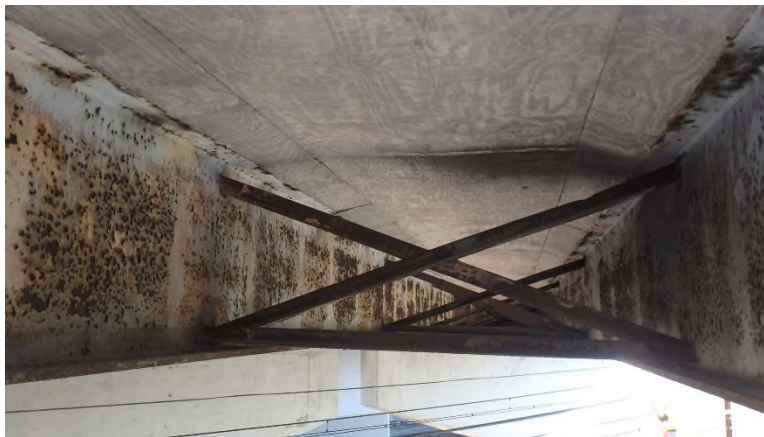
Photo SUP-23: Typical paint condition in Span 8 (Rust Grade 0)
