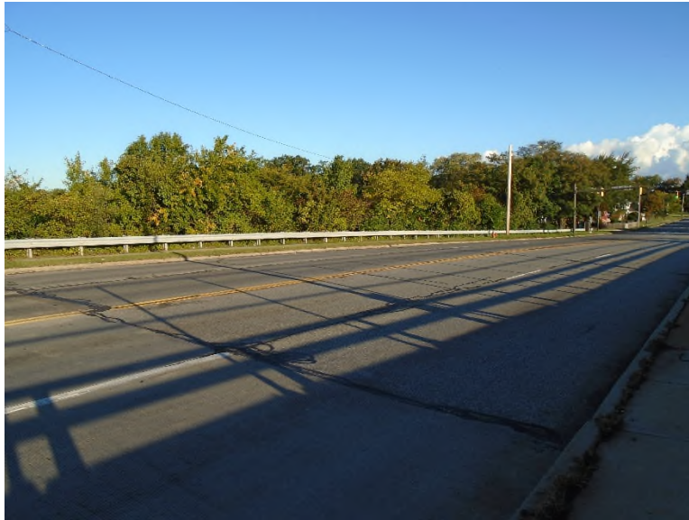
Photo APR-4: Forward Approach (looking north), cracks in asphalt wearing surface
