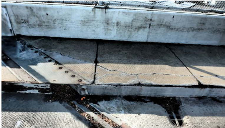
Photo DCK-13: Cracking and delaminations in left sidewalk at pier 5 expansion joint
