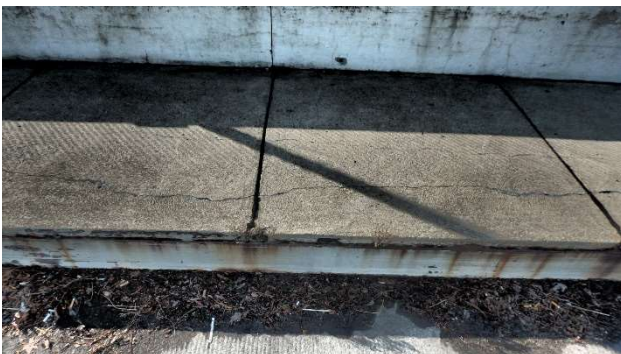
Photograph 321: Span 8 Deterioration @ diaphragm, bay 9, 2 south of pier 7
