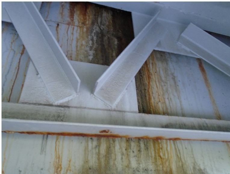
Photo SUB-8: Forward Backwall, cracking/leakage/rust staining
