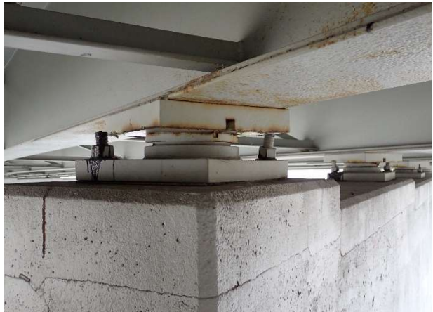
Photograph 140: Span 4 Beam 5 bearing - 2 anchor bolts pier 3
