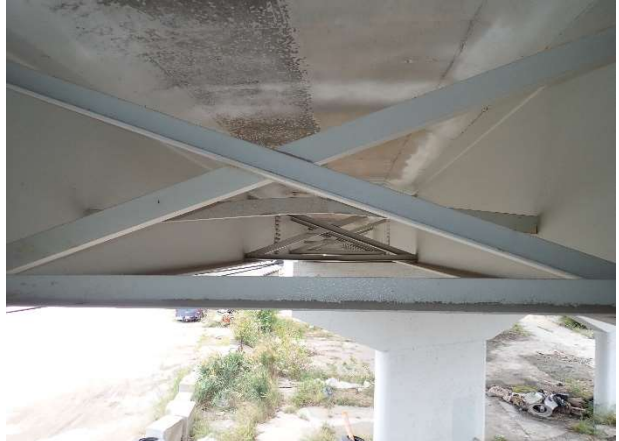
Photograph 182: Span 4 X-frame bay 9 bowed
