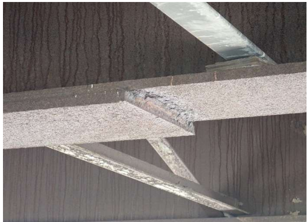
Photograph 340: Span 8 Moment weld pier 7 (3)
