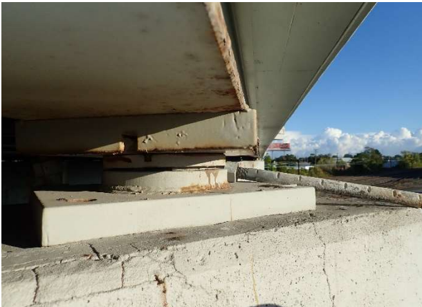
Photograph 151: Span 4 Beam 10 bearing - anchor bolt pier 4
