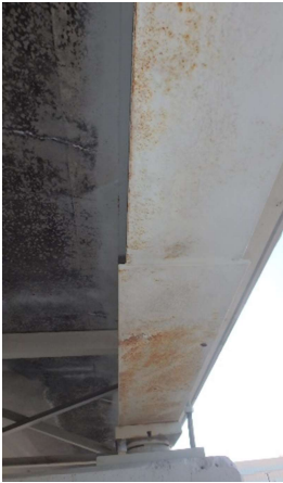
Photograph 93: Span 2 Rusting on bot
