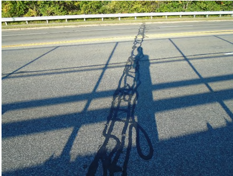
Photo APR-13: Forward Relief Joint
