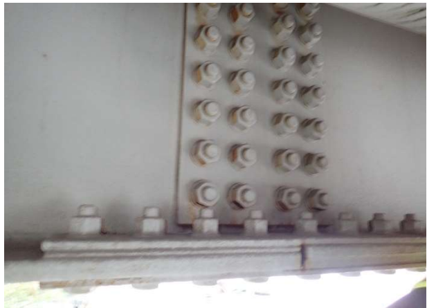
Photograph 178: Span 4 Splice lose bolts
