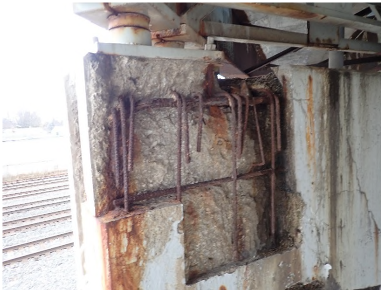
Photo SUB-22: Pier 5L, extensive spalling/deterioration at left end of cap.
