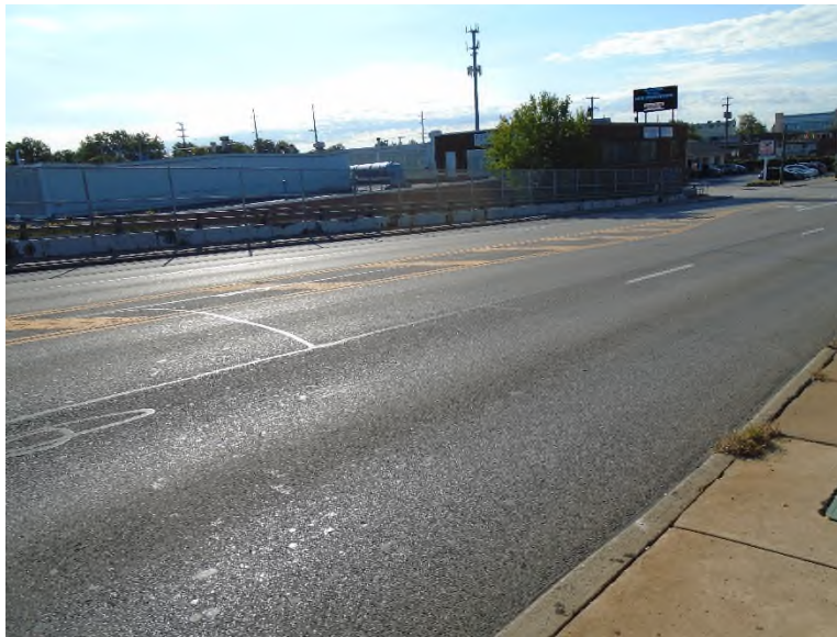
Photo APR-1: Rear Approach (looking south), minor cracks (sealed) in asphalt pavement
