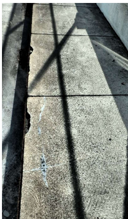
Photograph 365: Span 10 Longitudinal cracking in sidewalk minor spalls @ curb
