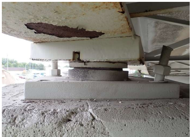
Photograph 150: Span 4 Beam 10 bearing - 1 of 2 bolts broke
