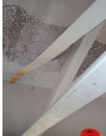
Photograph 158: Span 4 Broke x-frame 2
