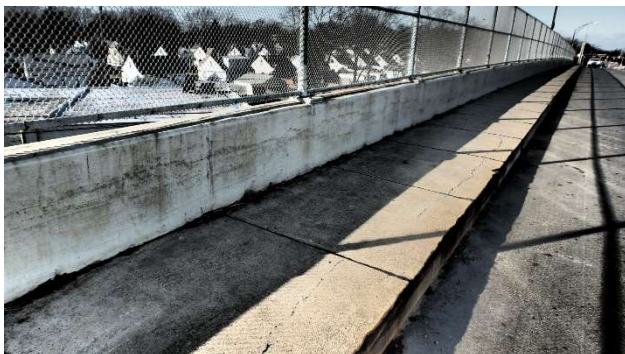
Photograph 279: Span 7 Sidewalk delam and spall 7'x1'
