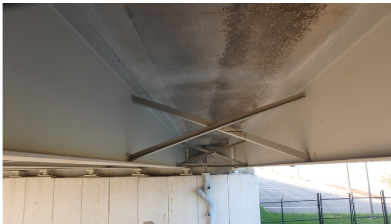
Photo SUP-11: Span 1, Bay 1, missing bottom intermediate x-frame angle
