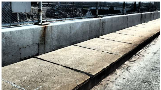
Photograph 280: Span 7 Sidewalk long cracks minor scaling
