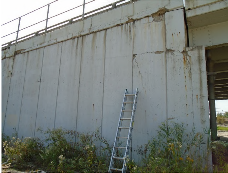
Photo SUB-9: Rear-right wingwall, cracking and minor delaminations/spalling
