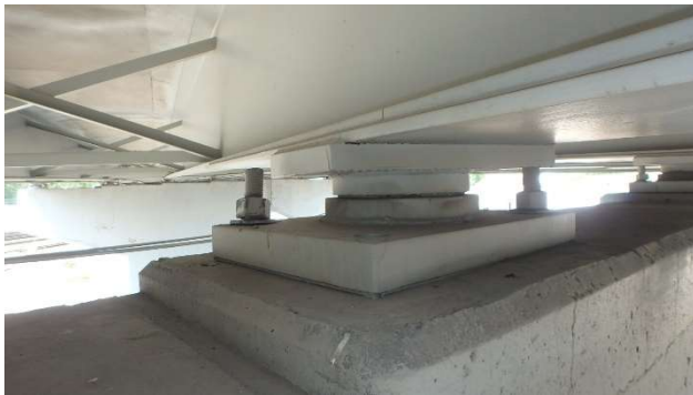
Photograph 55: Span 2 and 3 Beam 1 bearing on pier 2 facing N
