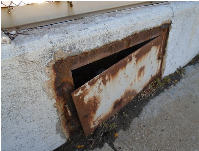
Photo UTL-2: Utility Access Panel, loose cover plate at forward-right approach
