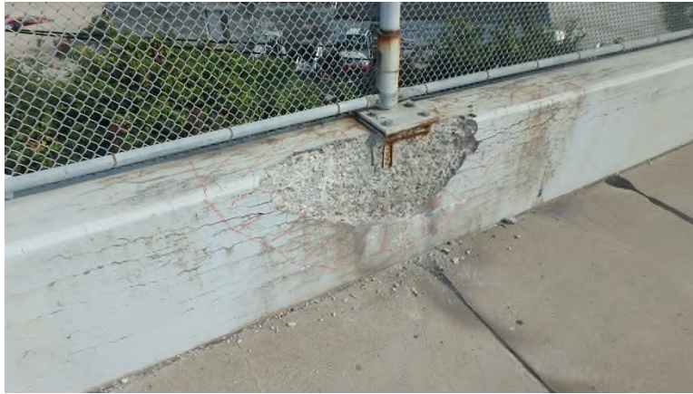
Photo DCK-17: Right Parapet, Saturated concrete/spall with exposed VPF anchor bolt
