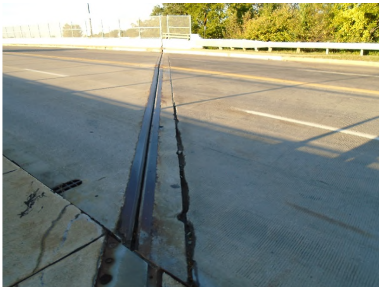
Photo SUB-6: Forward Backwall, minor chips/spalls along top
