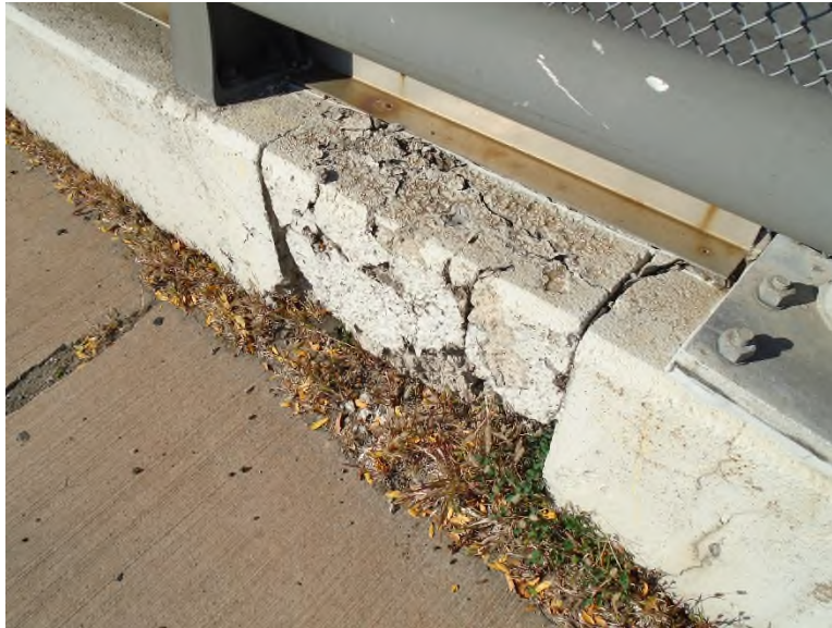
Photo APR-11: Missing bolts/screws in bottom closure angle
