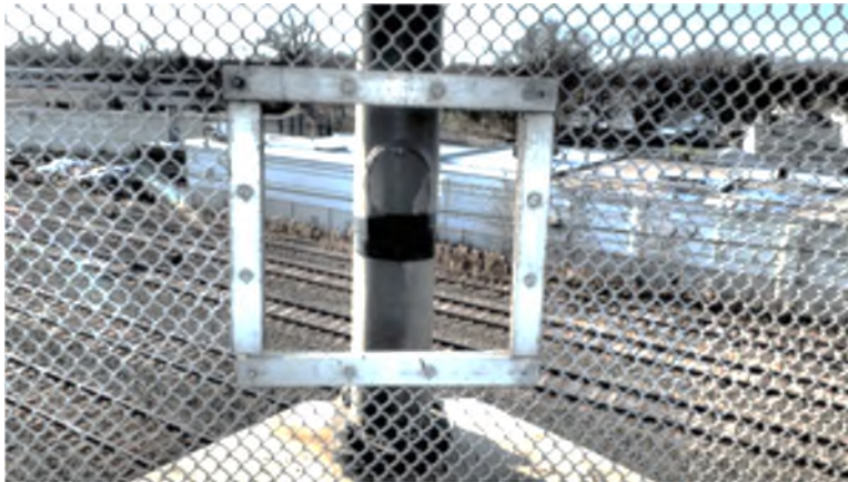
Photo DCK-22: Missing light pole access cover in vandal protection fence
