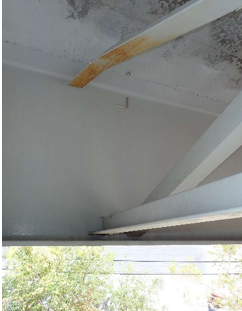
Photograph 157: Span 4 Broke x-frame
