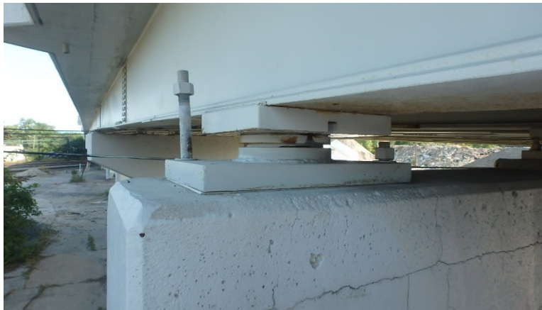
Photo SUP-15: Bearing 1/Pier 1, broke anchor bolt
