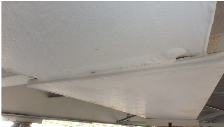
Photo SUP-25: Pack rust and small crack in transverse weld at end of moment plate in Span 1
