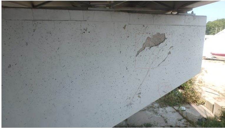
Photo SUB-18: Pier 2R, large spall and diagonal shear crack between Beams 9 and 10
