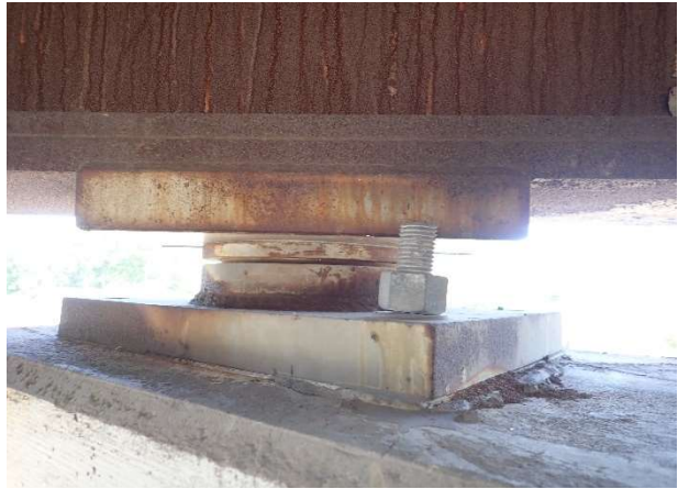
Photograph 310: Span 8 Beam 10 bearing pier 7 bent bolt
