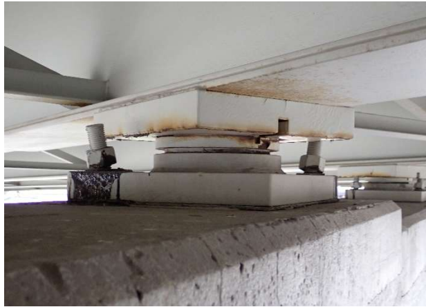
Photograph 154: Span 4 Beam bearing 4 - 2 anchor bolts pier 3
