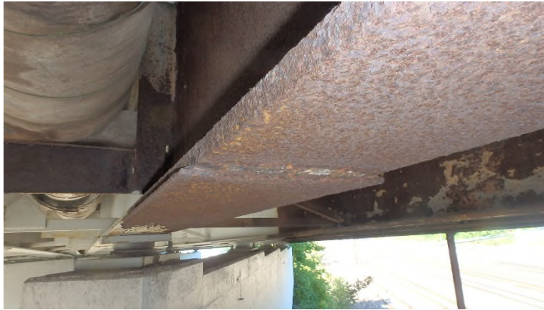
Photo SUP-24: Corrosion of bottom flange and moment plate in Span 8.
