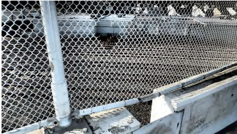
Photo DCK-21: Cut-out in chain link fence and kink in bottom rail at Pier 5 expansion joint.
