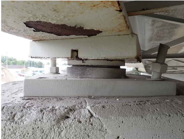
Photo SUP-16: Bearing 10/Pier 4, broken anchor bolt
