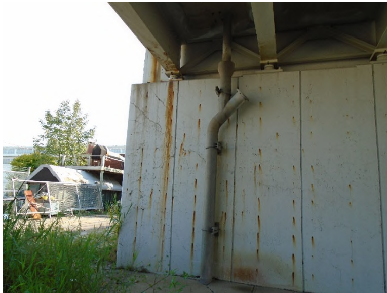
Photo SUB-1: Rear Abutment, cracking, leakage, and rust staining
