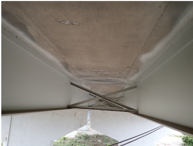
Photo DCK-2: Underside of deck, transverse cracks with leakage/leaching
