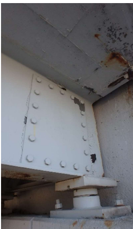
Photograph 23: Span 1 Beam 1 web retrofit typ
