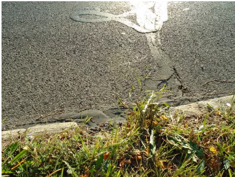
Photo APR-14: Forward Relief Joint, 1 foot length of curb is missing
