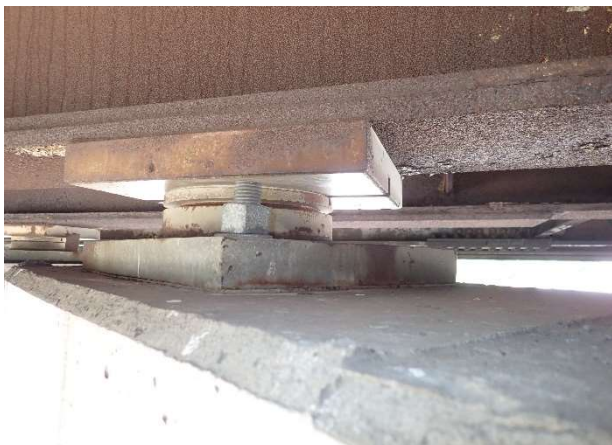
Photograph 317: Span 8 Bearing beam 5 missing bolt
