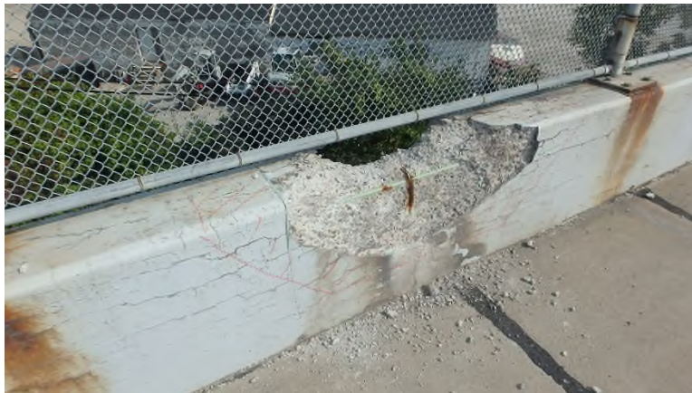
Photo DCK-18: Right Parapet, Saturated concrete/spall with exposed/corroded rebar.
