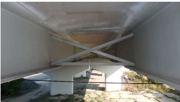
Photograph 69: Span 2 Bay 4 second interior cross frame broke and buckled
