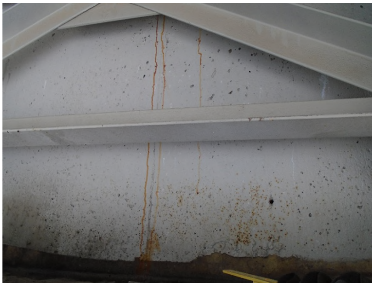
Photo DCK-25: South Expansion Joint, evidence of leakage onto backwall
