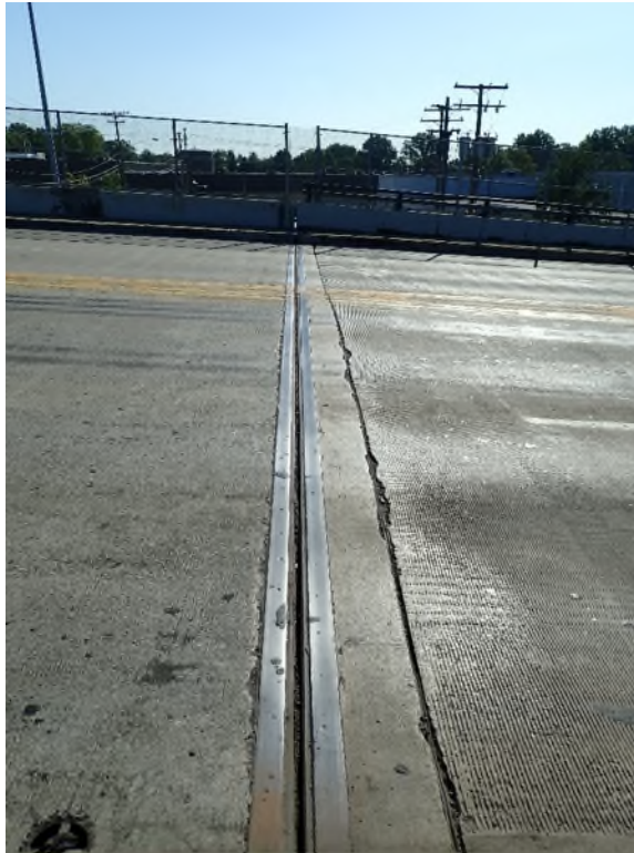
Photo APR-5: Rear Approach Slab, minor spalling along backwall joint
