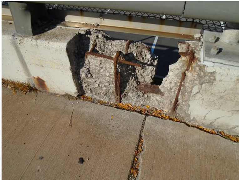
Photo APR-9: Approach Railing, concrete spalling/deterioration
