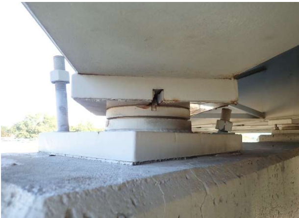
Photograph 135: Span 4 Beam 1 bearing - broke anchor pier 4
