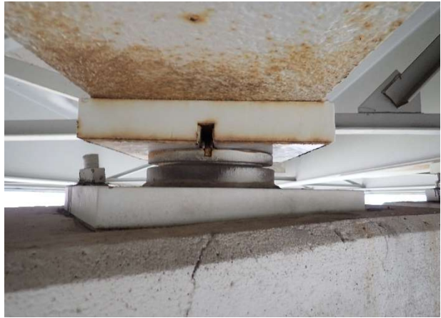
Photograph 142: Span 4 Beam 6 bearing - 1 anchor bolt pier 3
