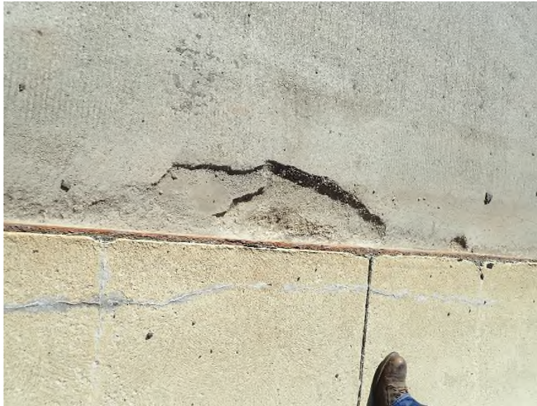
Photo DCK-9: Spall along right gutterline
