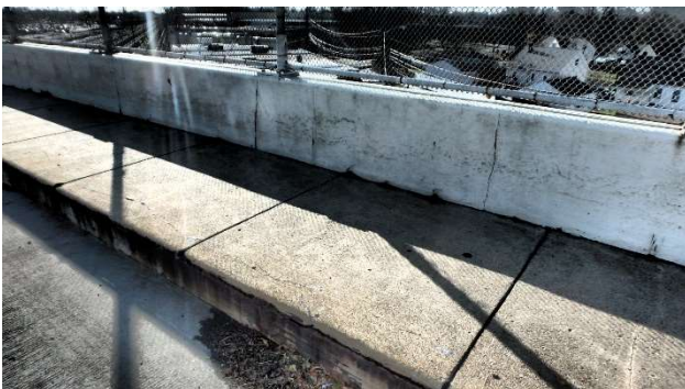
Photograph 357: Span 9 Long transverse crack in sidewalk
