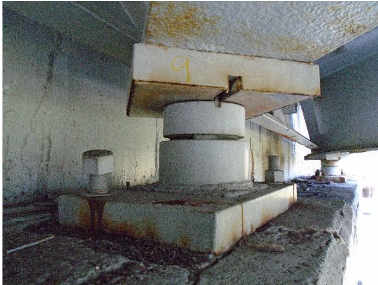
Photo SUP-19: - Bearing 9/Forward Abutment, light corrosion and loose nut
