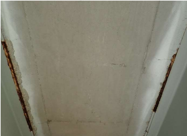
Photograph 111: Span 3 Bay 8 top moment plate rusted N
