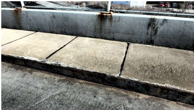
Photograph 349: Span 8 Sidewalk delam and spall 1'x1' (2)
