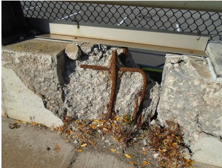
Photo APR-10: Approach Railing, concrete spalling/deterioration
