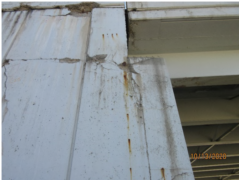
Photo SUB-2: Rear Abutment, cracking and spalling at right end face.
