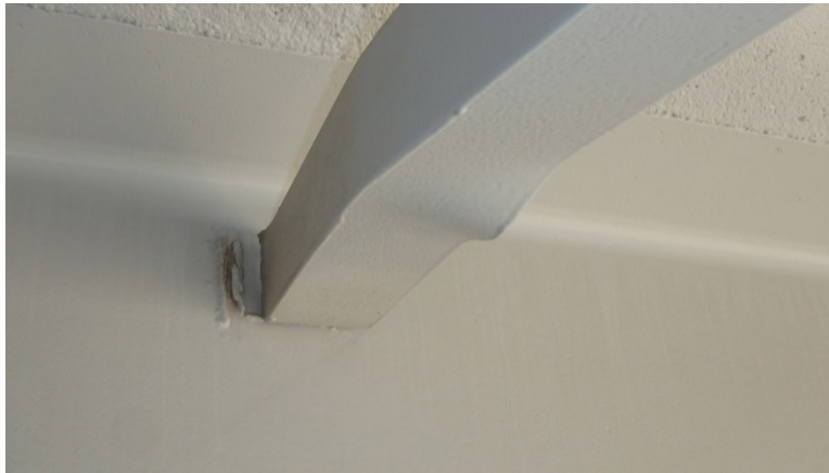
Photo SUP-10: Span 1, Bay 3, broken weld/buckled diagonal x-frame frame member
