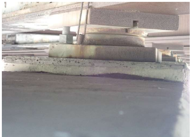
Photograph 312: Span 8 Bearing @ beam 8
