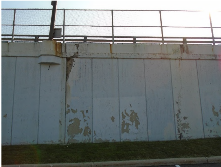
Photo SUB-12: Rear-left retaining wall, cracking and minor delaminations/spalling
