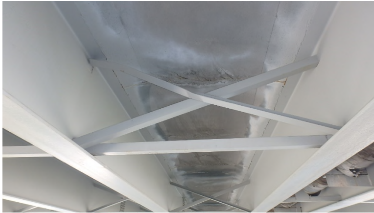
Photo SUP-12: Span 2, Bay 4, broken weld/buckled intermediate x-frame member
