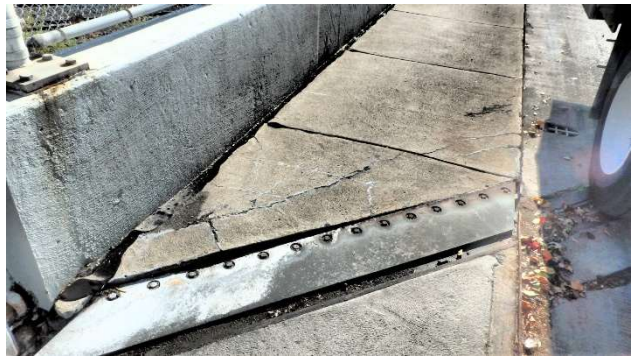
Photograph 368: Span 10 Sidewalk delam and spall 5'x1'
