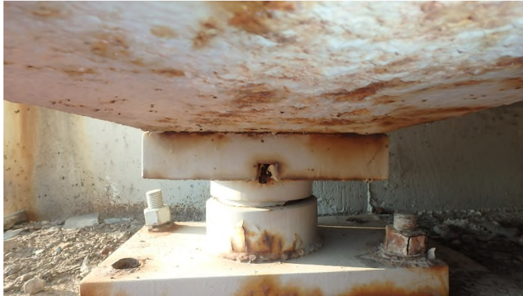
Photo SUP-14: Bearing 10/Rear Abutment, corrosion of bearing
