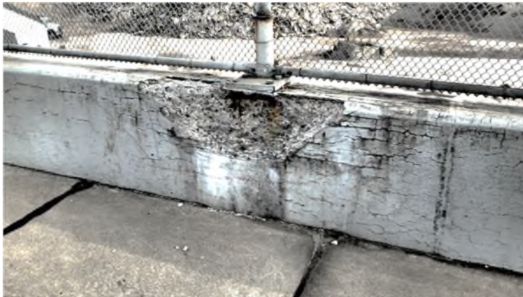
Photo DCK-20: Right Parapet, Saturated concrete/spall with exposed VPF anchor bolt
