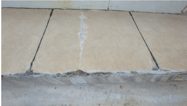
Photo DCK-11: Chipping and spalling of sidewalk behind curb plate (typ.)
