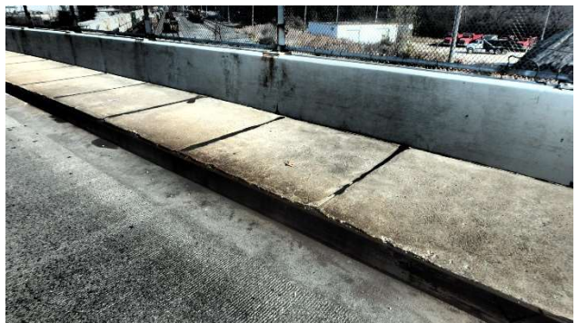
Photograph 262: Span 6 Sidewalk delam and spall 3'x1'
