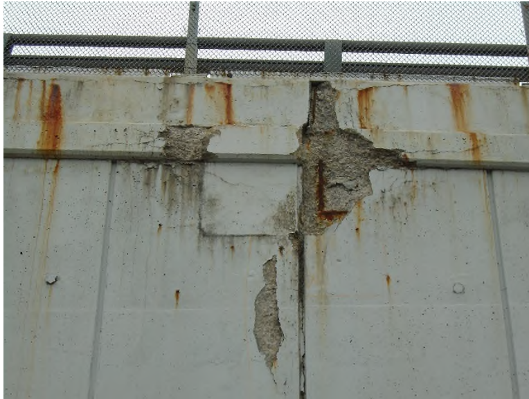
Photo SUB-14: Forward-right retaining wall, delaminations/spalls near top of wall
