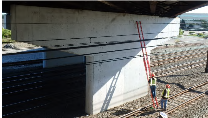
Photo EQP-2: Inspection access using extension ladders
