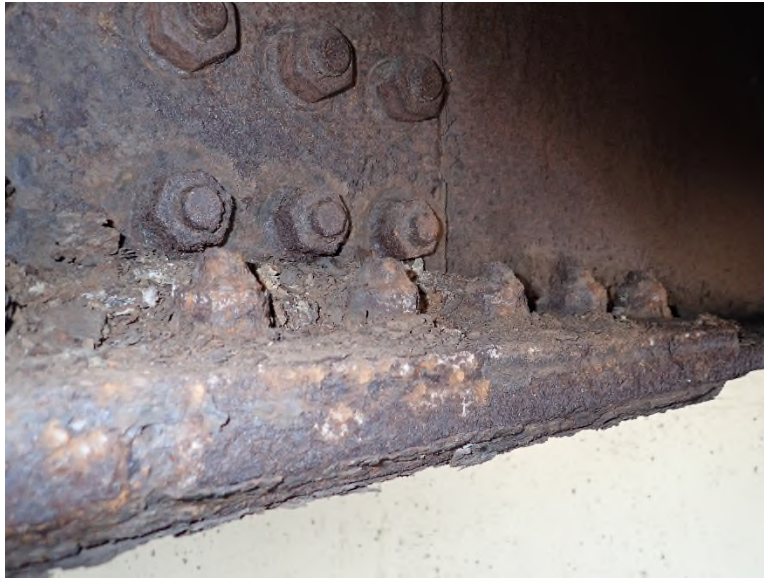
Photo SUP-8: Beam 6/Span 7, advanced corrosion/pack rust at bottom flange field splices
