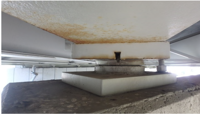
Photo SUP-18: - Bearing 6/Pier 9, missing anchor bolt
