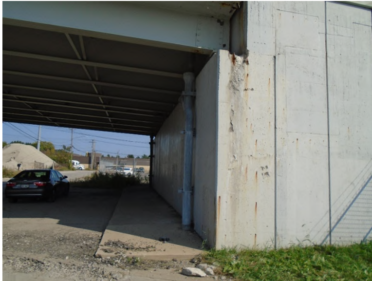
Photo SUB-3: Rear Abutment, cracking and spalling at left end face.
