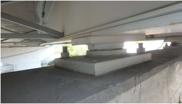
Photograph 61: Span 2 and 3 Beam 7 bearing on pier 2 facing N
