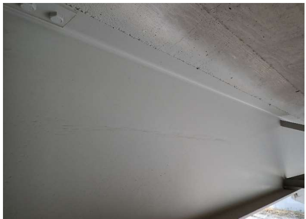
Photograph 162: Span 4 Gouge in beam
