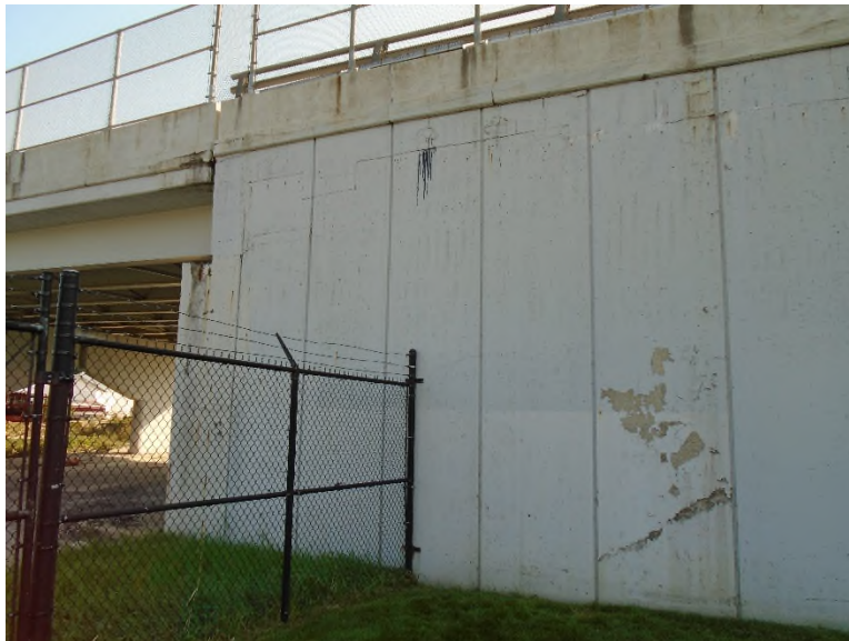
Photo SUB-11: Rear-left wingwall, minor cracking and delaminations
