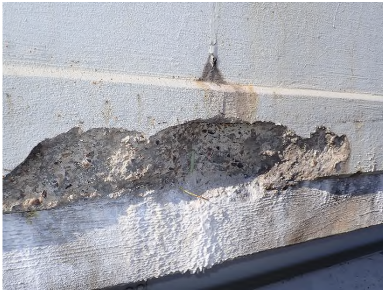
Photo DCK-8: Spall in parapet coping
