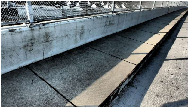
Photograph 211: Span 5 Sidewalk delam and spall 3'x1'
