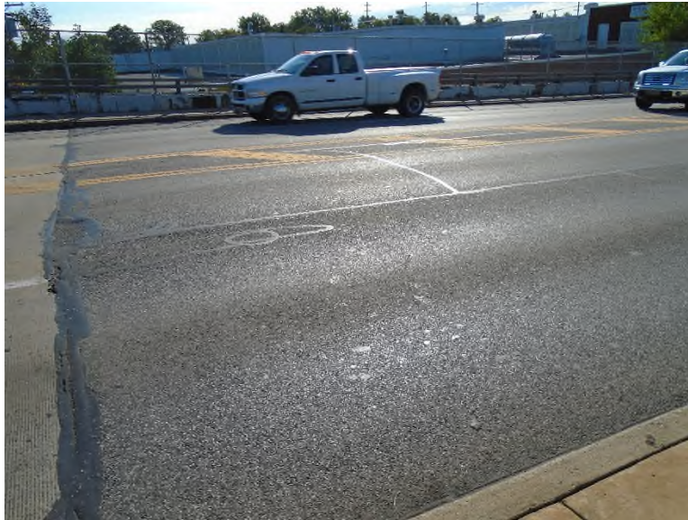
Photo APR-2: Rear Approach (looking east), minor potholes along asphalt/concrete pavement joint
