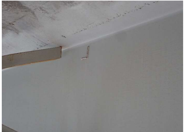
Photograph 160: Span 4 Broken x-frame
