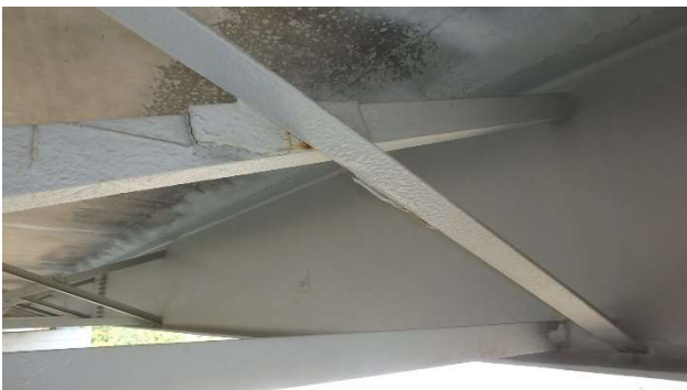
Photograph 75: Span 2 Bay 9 fifth interior x frame deterioration
