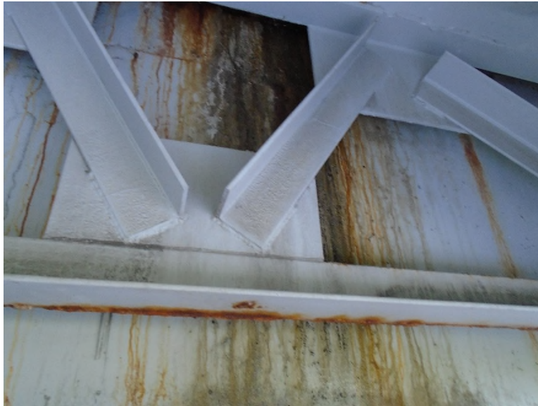
Photo DCK-27: North Expansion Joint, evidence of leakage onto backwall
