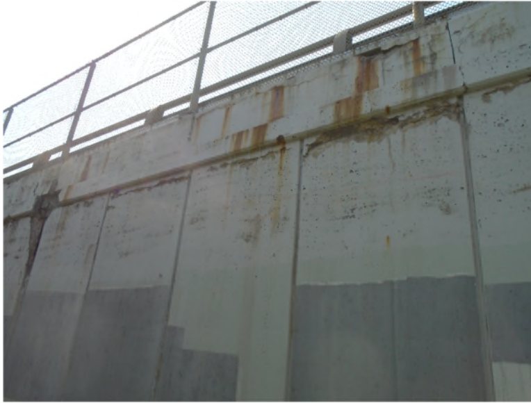
Photo SUB-10: Rear-right retaining wall, cracking and minor delaminations/spalling
