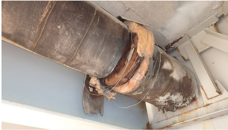
Photo UTL-3: Exposed water-line insulation
