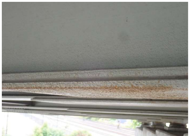
Photograph 174: Span 4 Pitted moment - side
