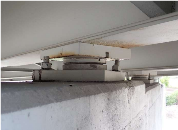
Photograph 153: Span 4 Beam bearing 3 - 2 anchor bolts pier 3
