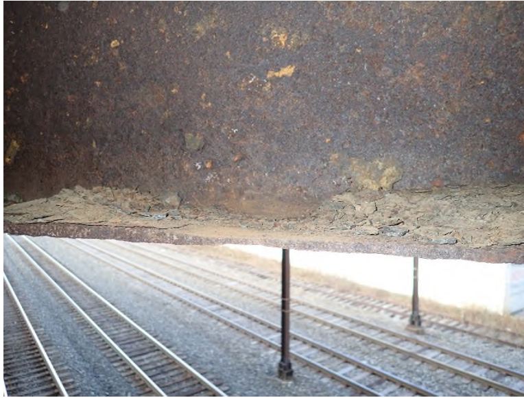
Photo SUP-6: Beam 6/Span 7, advanced corrosion/section loss at lower flange
