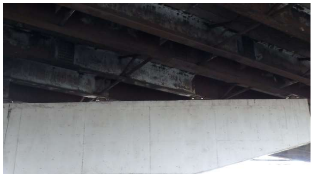
Photograph 250: Span 6 Parapet spall and deterioration 1'x3'
