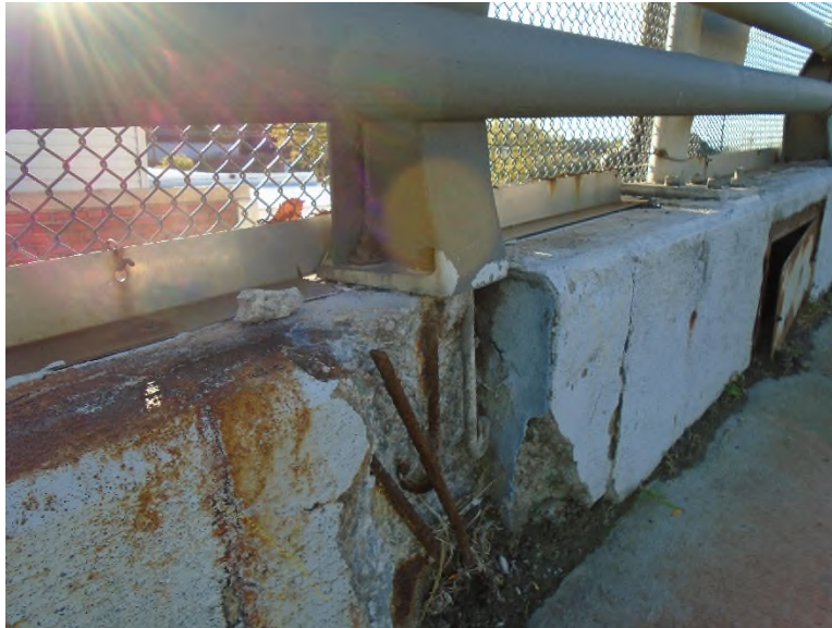
Photo APR-8: Approach Railing, concrete spalling/deterioration
