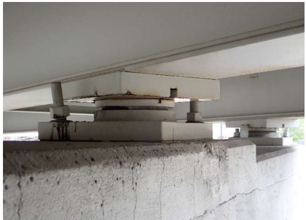
Photograph 136: Span 4 beam 2 bearing - 2 anchor bolts pier 3
