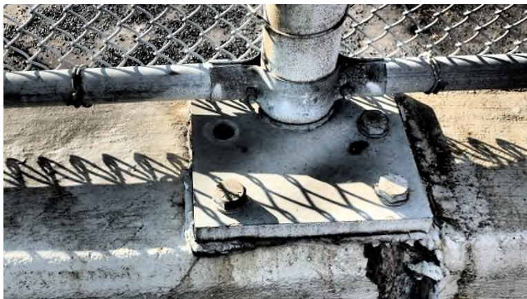
Photo DCK-23: Missing anchor bolt in fence base plate.
