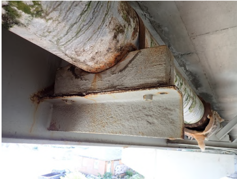
Photo UTL-4: Exposed water-line insulation and corroded support angle.
