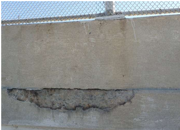
Photograph 177: Span 4 Spall W
