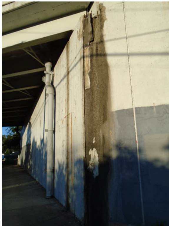
Photo SUB-4: Forward Abutment, leakage and spalling at right end face.
