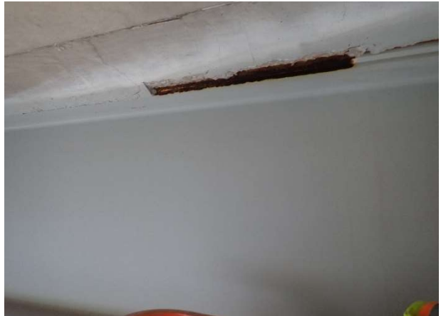
Photograph 112: Span 3 Bay 8 top moment plate rusted S
