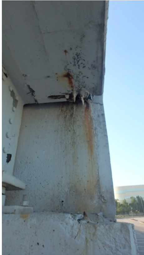
Photo DCK-26: South Expansion Joint, evidence of leakage onto backwall
