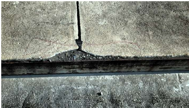
Photograph 265: Span 6 Sidewalk parapet long cracks in sidewalk
