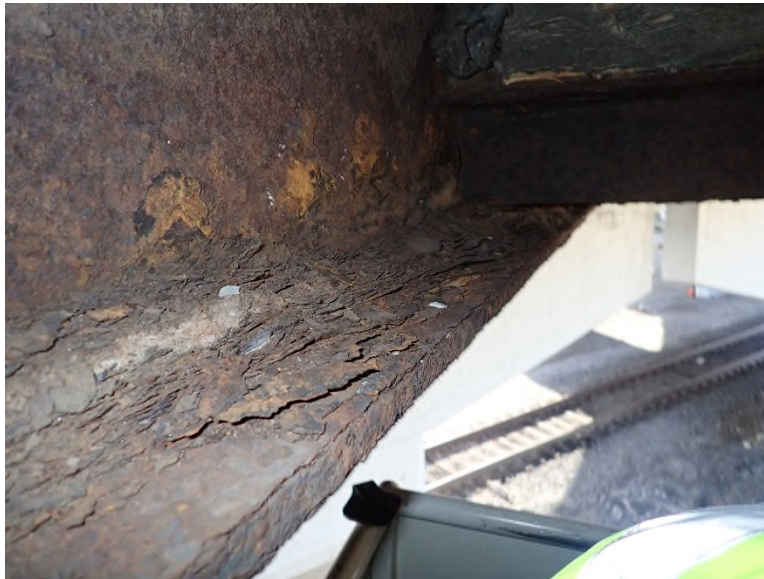
Photo SUP-7: Beam 5/Span 7, advanced corrosion/pack rust at lower flange
