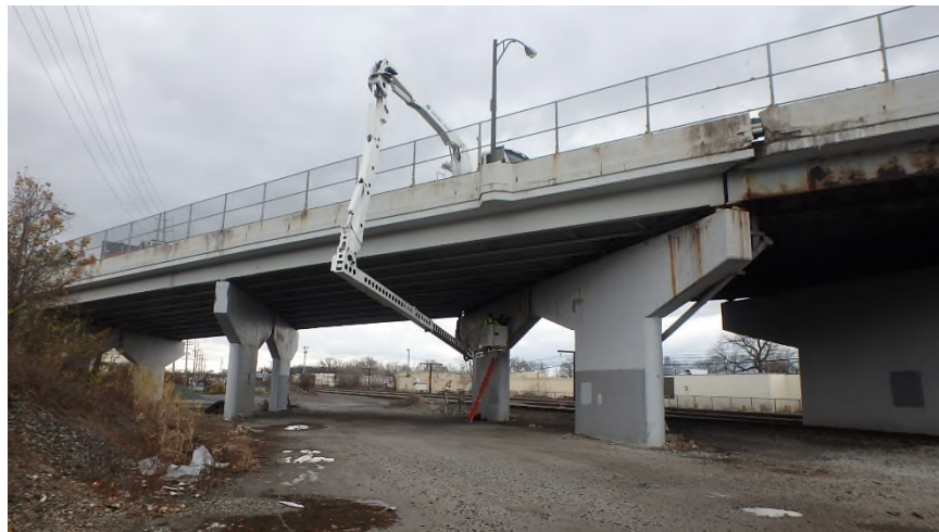
Photo EQP-1: Inspection access using underbridge inspection vehicle (Snooper)
