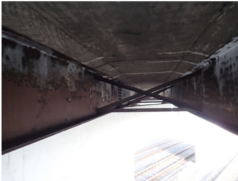
Photo SUP-21: Typical paint condition in Span 6 (Rust Grade 0).
