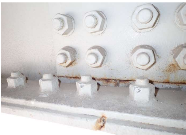
Photograph 179: Span 4 Splice lose bolts 2
