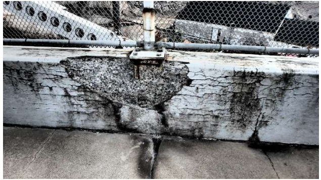
Photograph 170: Span 4 Parapet spall deterioration 4'x2'x1'
