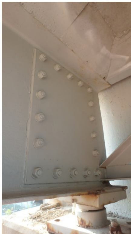
Photo SUP-2: Span 1, Beam 10 web plate repairs
