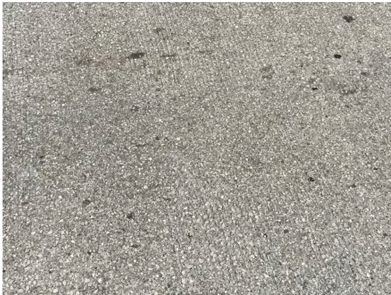
Photo DCK-10: Minor transverse crack and wearing/abrasion in wheel path
