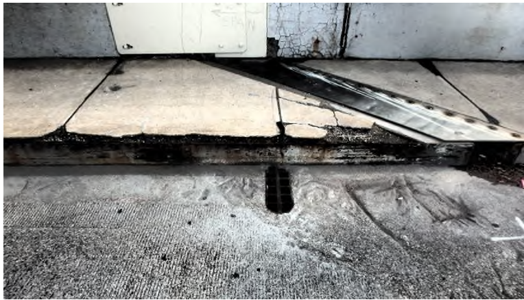
Photo DCK-14: Spalling in right sidewalk at Pier 5 expansion joint.
