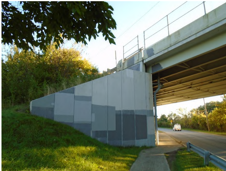
Photo SUB-15: Forward-left wingwall, no problems
