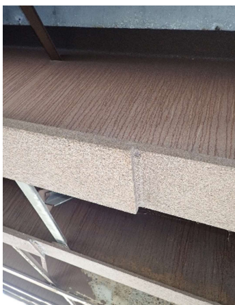
Photograph 341: Span 8 Moment weld pier 7
