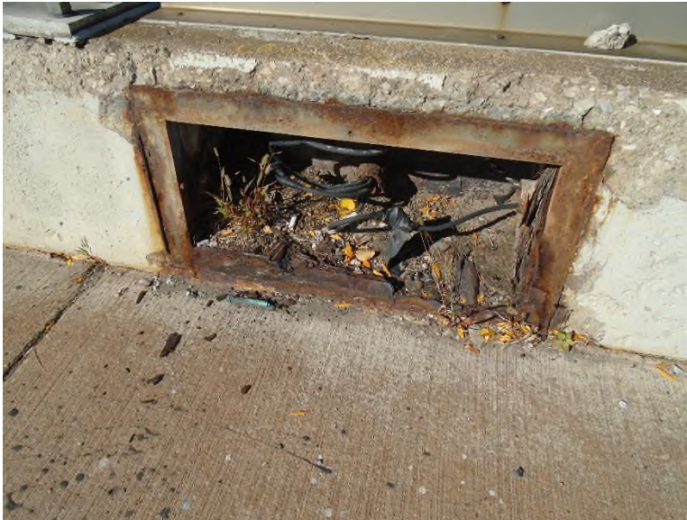
Photo UTL-1: Utility Access Panel, missing cover plate and exposed wires (typ. at 3 locations)
