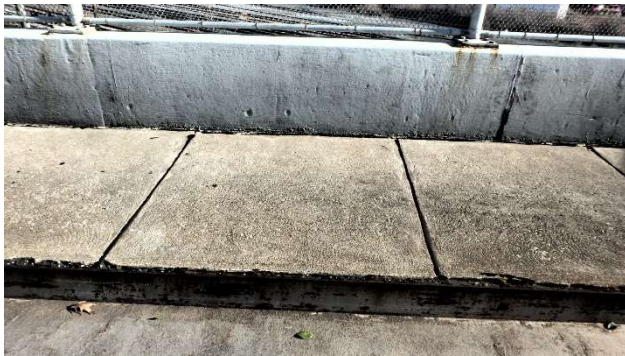
Photograph 367: Span 10 Parapet wall cracking missing hardware @ VPF opening
