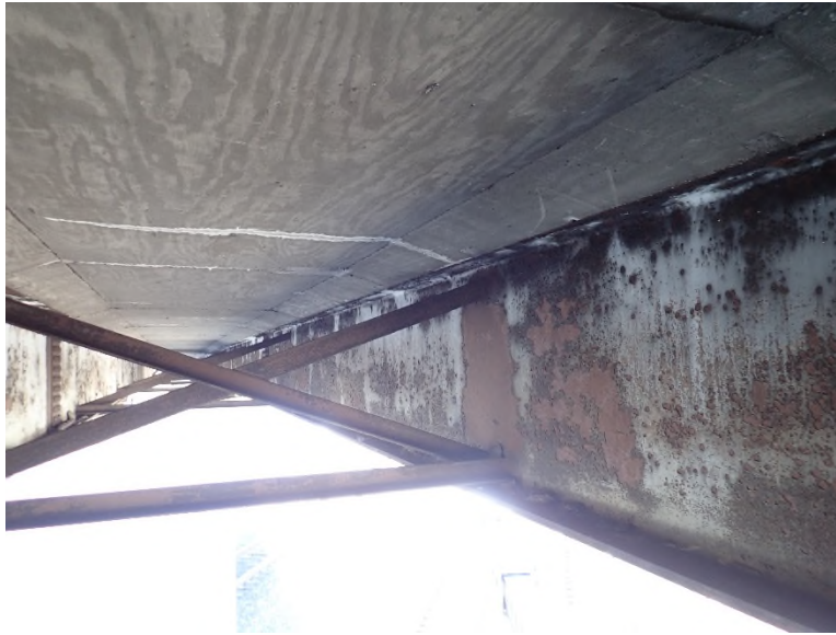
Photo SUP-22: Typical paint condition in Span 7 (Rust Grade 0)
