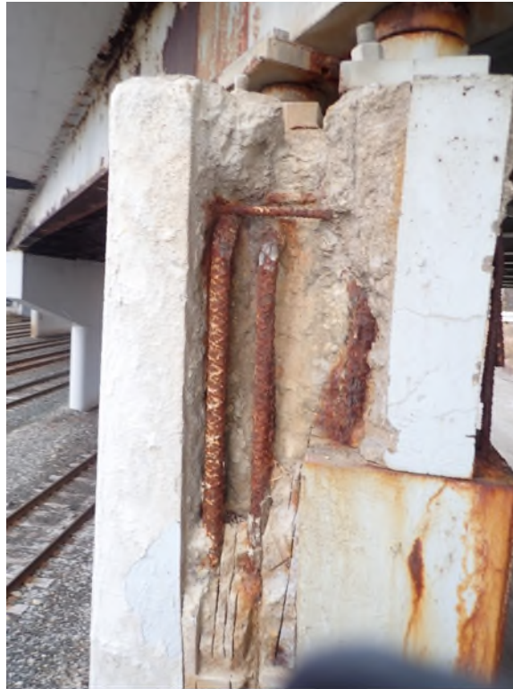
Photo SUB-21: Pier 5L, extensive spalling/deterioration at left end of cap
