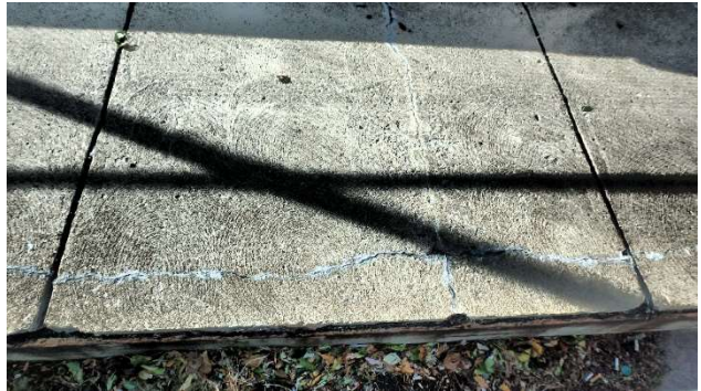
Photograph 362: Span 9 Sidewalk delam and spall 2'x1'
