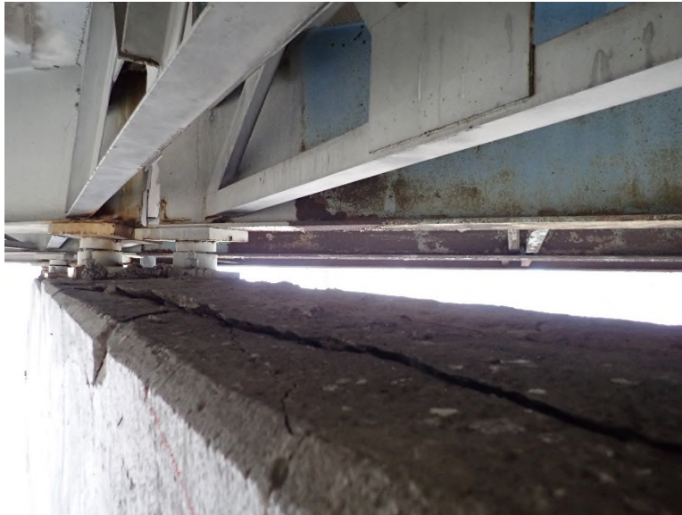
Photo SUB-23: Pier 5L, large crack/delamination in pier seat.
