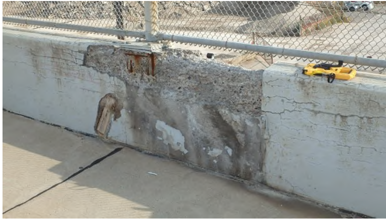
Photo DCK-19: Right Parapet, Saturated concrete/spall with exposed VPF anchor bolts
