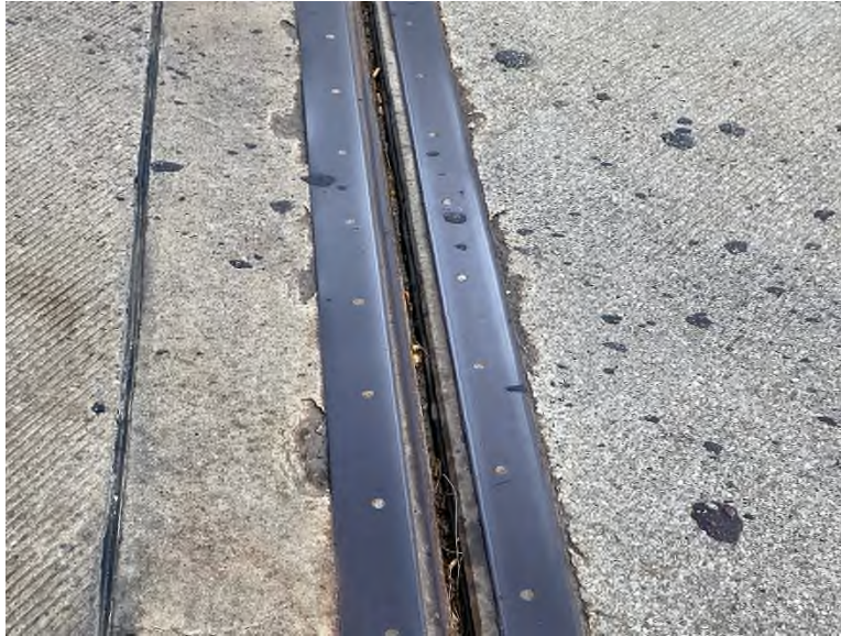
Photo DCK-24: Dirt and debris in elastomeric strip seal
