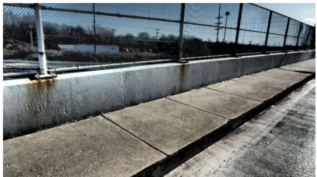
Photograph 364: Span 10 Long transverse crack in sidewalk
