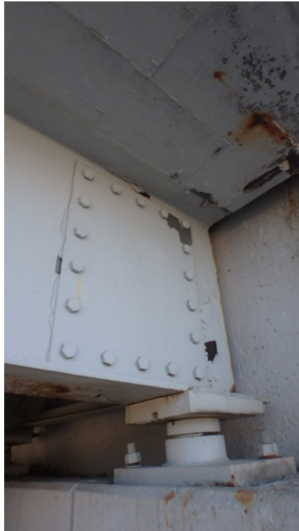
Photo SUP-1: Span 1, Beam 1 web plate repairs
