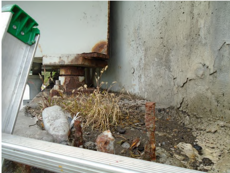
Photo SUB-5: Forward Abutment, spalling/exposed rebar at right end of beam seat
