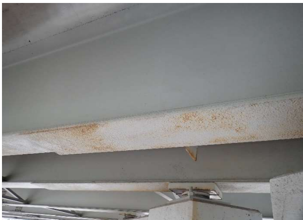
Photograph 173: Span 4 Pitted moment - bottom
