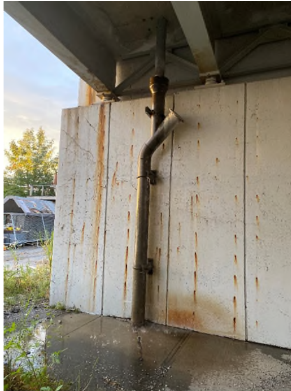
Photo DCK-28: Overflowing downspout at rear-right corner
