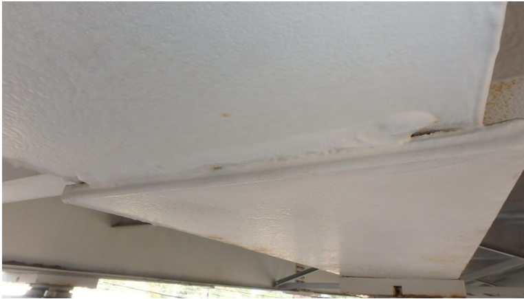
Photo SUP-3: Span 1, Beam 2, transverse weld at end of moment plate
