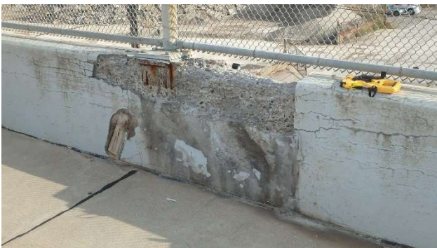
Photograph 45: Span 1 Parapet map cracking @ SE corner
