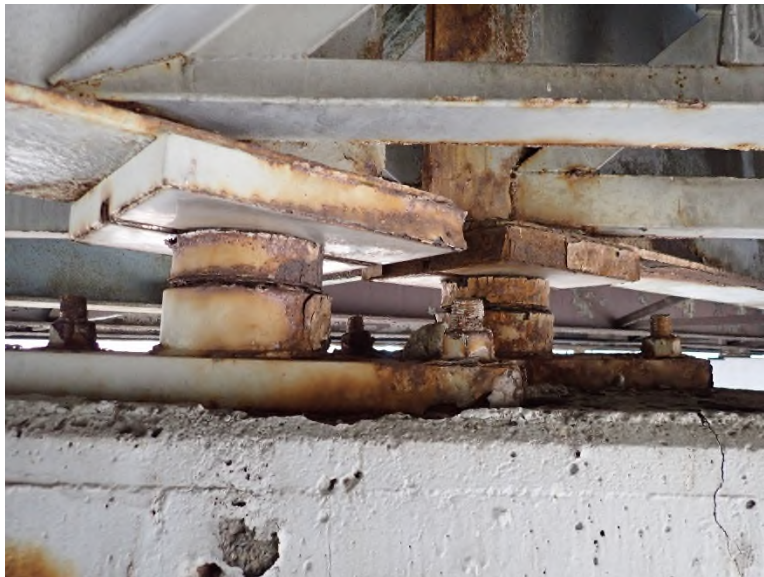
Photo SUP-17: Bearing 5/Pier 5, corrosion/pack rust
