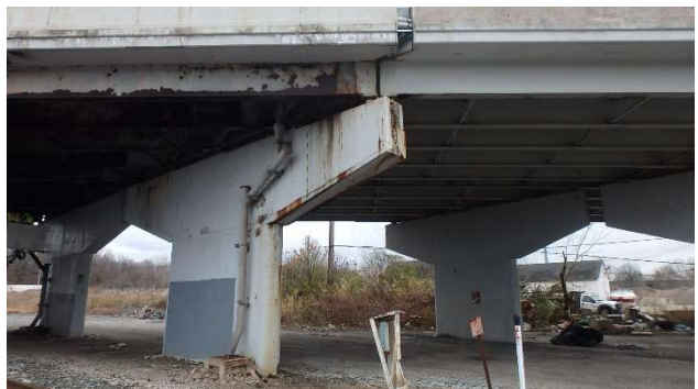
Photograph 238: Span 6 Long diagonal cracks near exp joint
