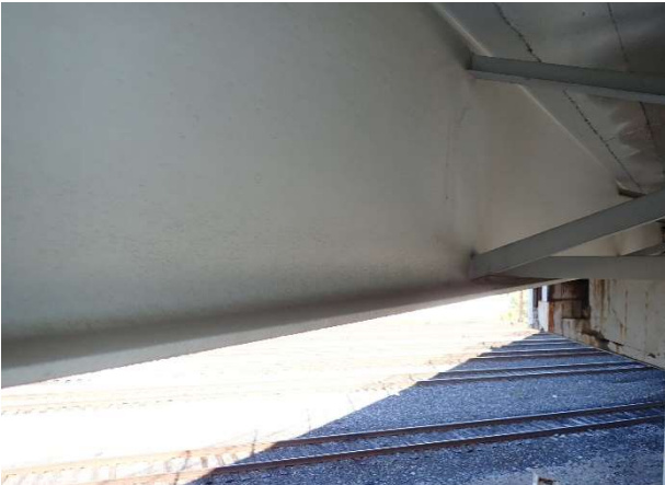
Photograph 183: Span 5 Beam 2 pitted flange
