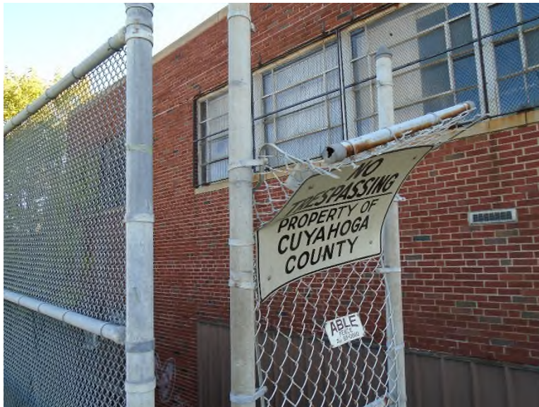
Photo APR-12: Damaged gate at south end of rear-right approach railing.
