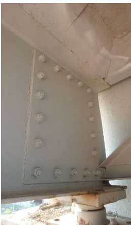
Photograph 35: Span 1 Beam 10 web retrofit typ
