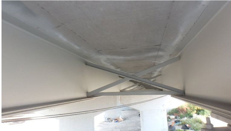
Photo SUP-20: Typical paint condition in Span 2 (Rust Grade 10)
