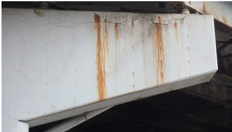
Photo SUB-19: Pier 5R, cracking/delaminations/rust staining at right end of cap
