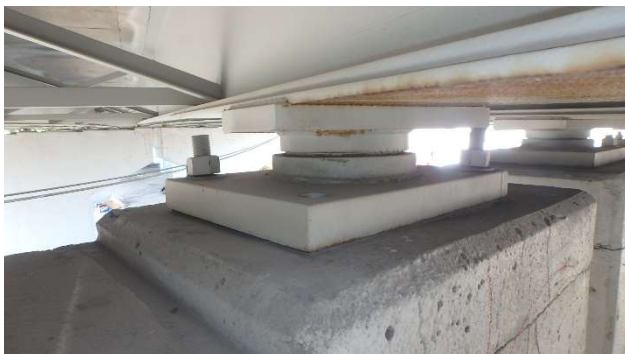
Photograph 57: Span 2 and 3 Beam 3 bearing on pier 2 facing N
