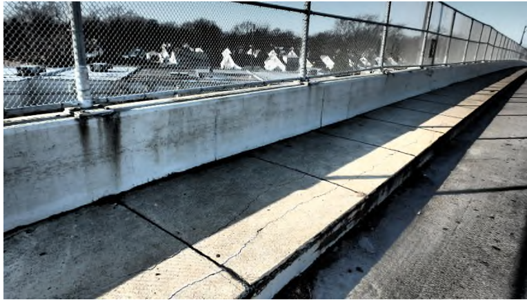
Photo DCK-15: Longitudinal cracking in left sidewalk (typical along length)
