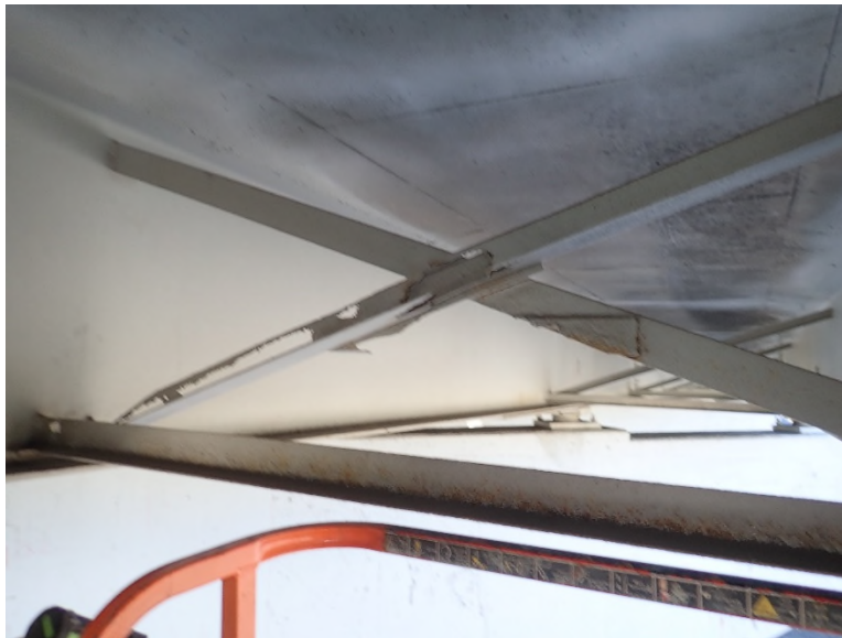
Photo SUP-13: Span 5, Bay 1, deteriorated x-frame
