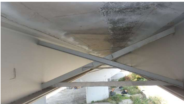
Photograph 111: Span 3 Bay 8 top moment plate rusted N
