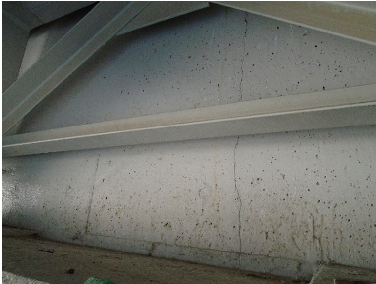
Photo SUB-7: Rear Backwall, minor vertical cracks
