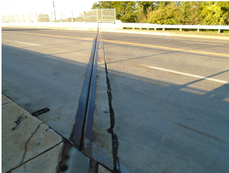
Photo APR-6: Forward Approach Slab, 3" wide x 16' long spall along backwall joint
