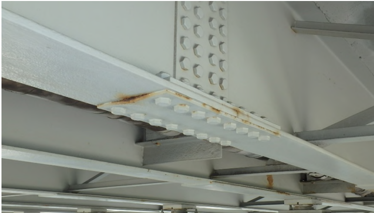
Photo SUP-4: Span 2, pack rust at bottom flange bolted field splice
