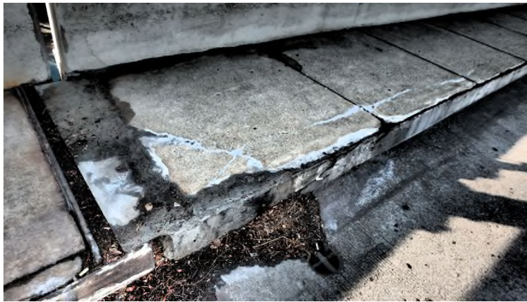
Photo DCK-12: Cracking and delaminations in left sidewalk at rear expansion joint
