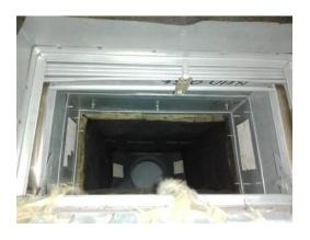
**Picture of Damper in Closed Position**
