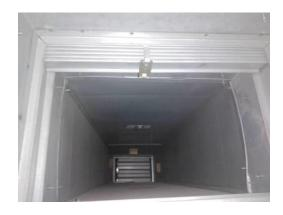
**Picture of Damper in Closed Position**
