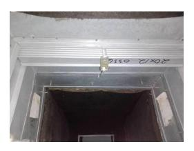
**Picture of Damper in Closed Position**
