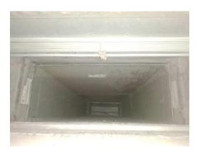
**Picture of Damper in Closed Position**
