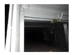
**Picture of Damper in Closed Position**
