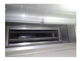
**Picture of Damper in Closed Position**
