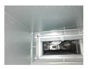
**Picture of Damper in Closed Position**
