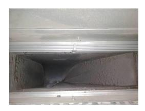
**Picture of Damper in Closed Position**
