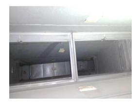
**Picture of Damper in Closed Position**
