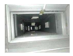
**Picture of Damper in Closed Position**
