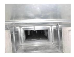
**Picture of Damper in Closed Position**
