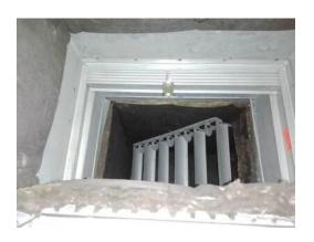
**Picture of Damper in Closed Position**
