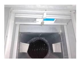
**Picture of Damper in Closed Position**
