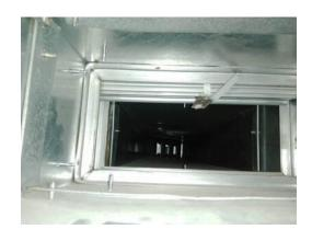
**Picture of Damper in Closed Position**
