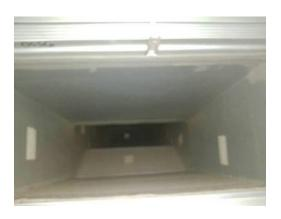
**Picture of Damper in Closed Position**
