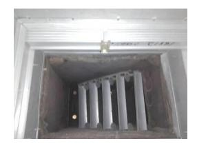
**Picture of Damper in Closed Position**
