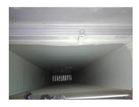
**Picture of Damper in Closed Position**
