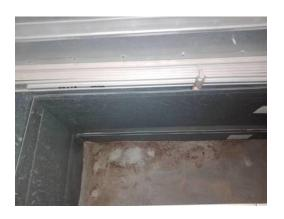
**Picture of Damper in Closed Position**
