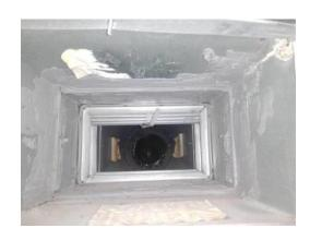
**Picture of Damper in Closed Position**
