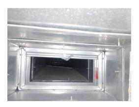
**Picture of Damper in Closed Position**
