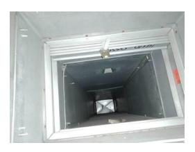
**Picture of Damper in Closed Position**
