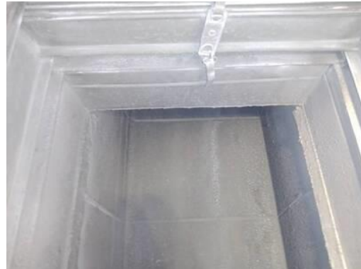
Picture of Damper in Closed Position
