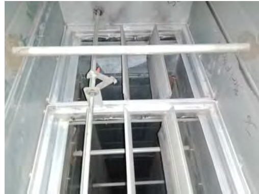
Picture of Damper in Closed Position
