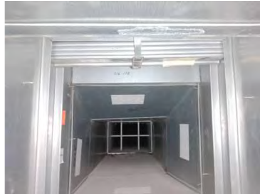
Picture of Damper in Closed Position
