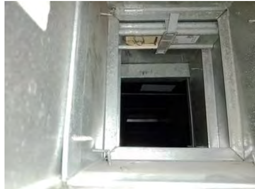
Picture of Damper in Closed Position
