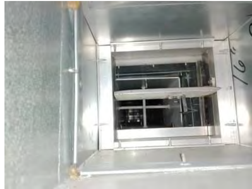
Picture of Damper in Closed Position
