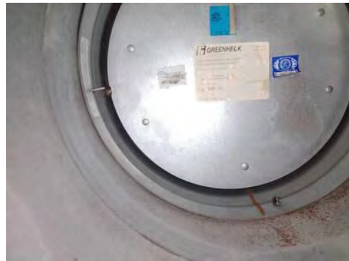
Picture of Damper I.D. Label
