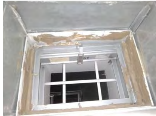
Picture of Damper in Closed Position
