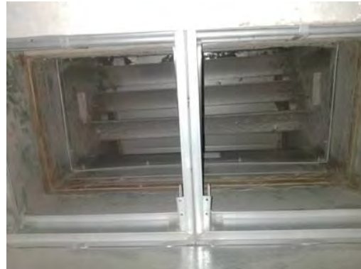
Picture of Damper in Closed Position
