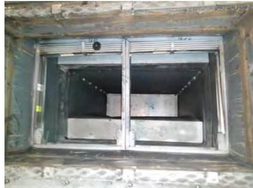
Picture of Damper in Closed Position
