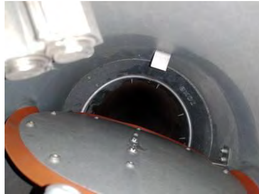
Picture of Damper in Closed Position
