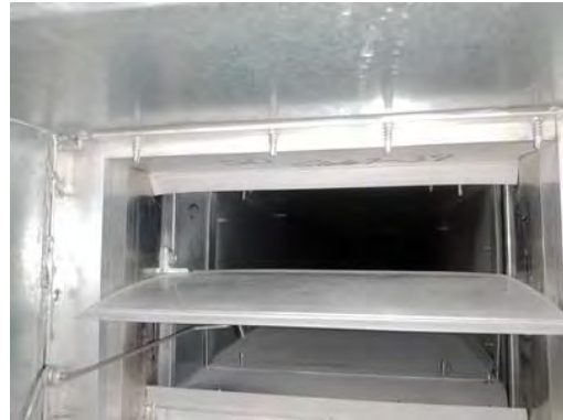
Picture of Damper in Closed Position
