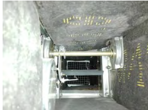
Picture of Damper in Closed Position
