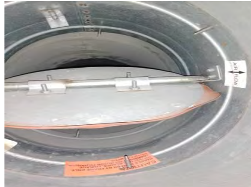
Picture of Damper in Closed Position
