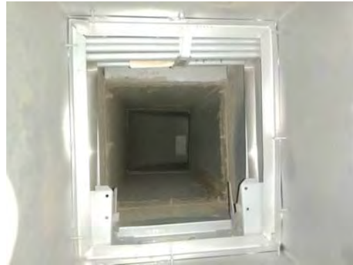
Picture of Damper in Closed Position
