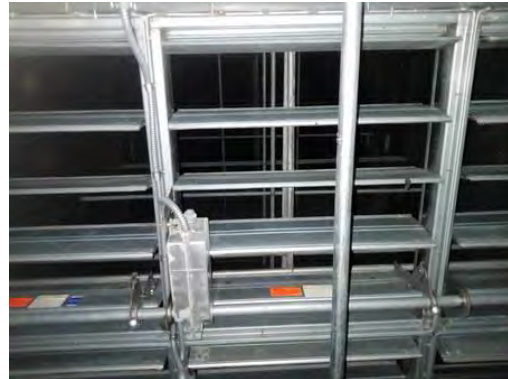
Picture of Damper in Closed Position
