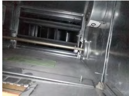
Picture of Damper in Closed Position
