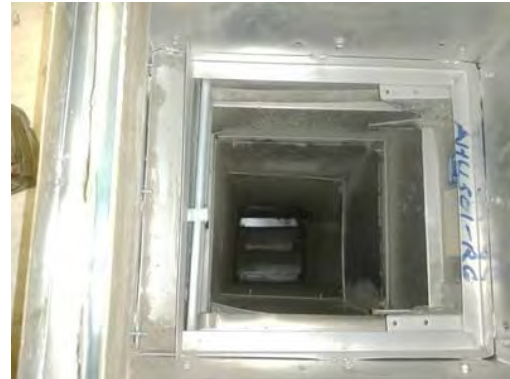
Picture of Damper in Closed Position
