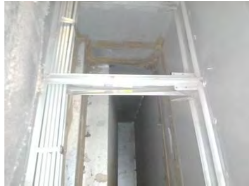
Picture of Damper in Closed Position
