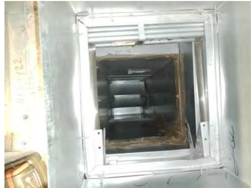
Picture of Damper in Closed Position
