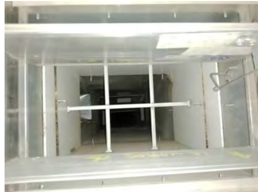
Picture of Damper in Closed Position
