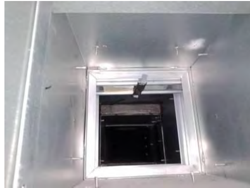
Picture of Damper in Closed Position
