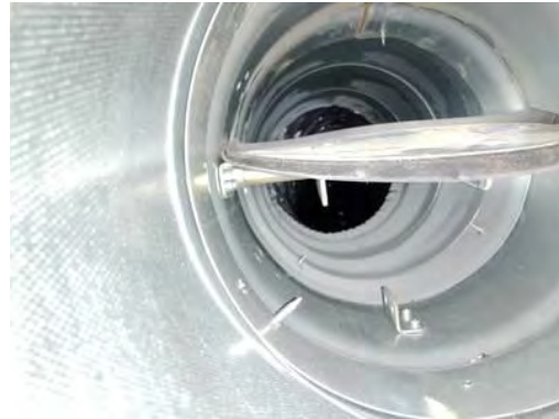
Picture of Damper in Closed Position
