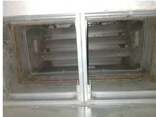
Picture of Damper in Closed Position
