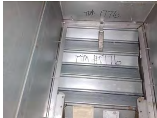
Picture of Damper I.D. Label
