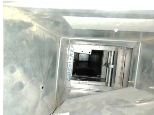
Picture of Damper in Closed Position
