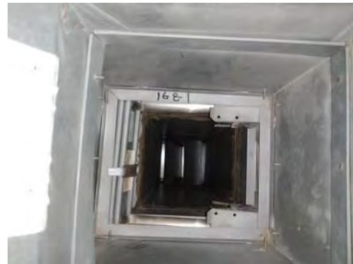
Picture of Damper in Closed Position
