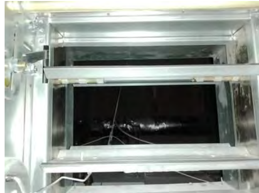
Picture of Damper in Closed Position
