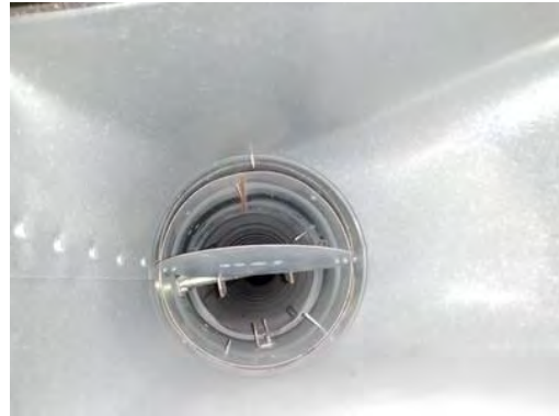
Picture of Damper in Closed Position
