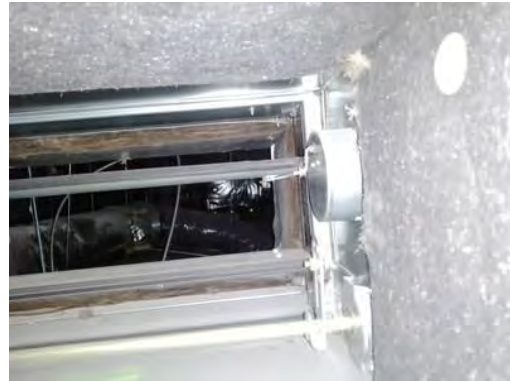
Picture of Damper in Closed Position
