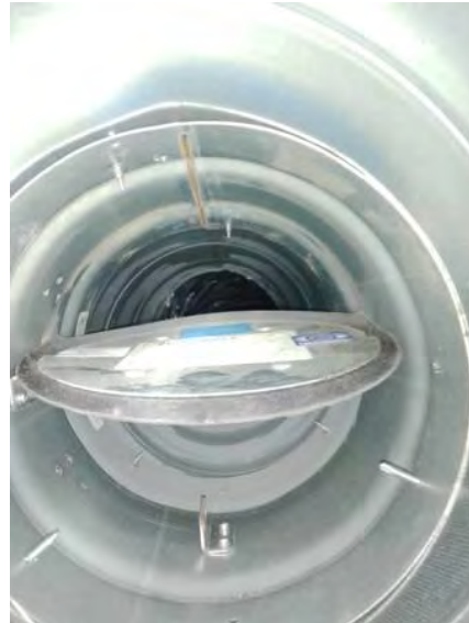
Interior Picture of Damper
