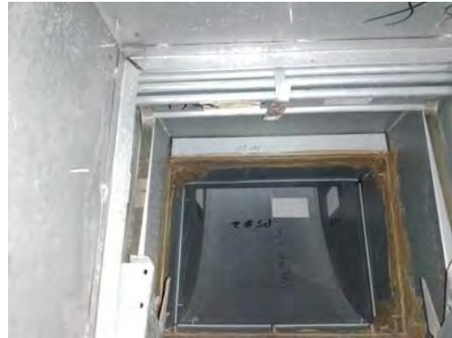
Picture of Damper in Closed Position
