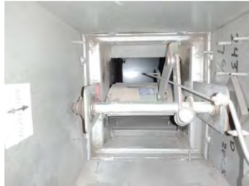
Picture of Damper in Closed Position
