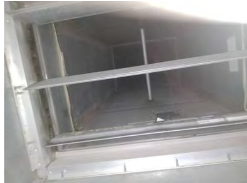
Picture of Damper in Closed Position
