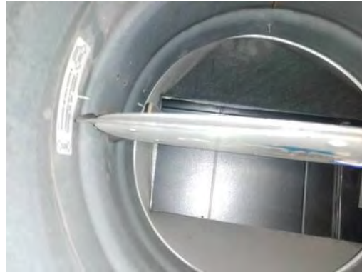
Picture of Damper in Closed Position
