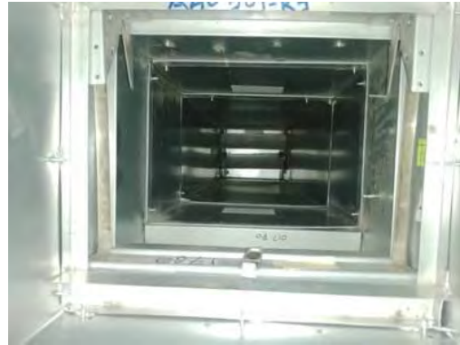
Picture of Damper in Closed Position
