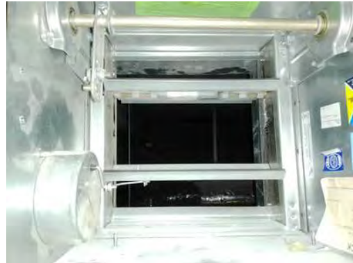
Picture of Damper in Closed Position
