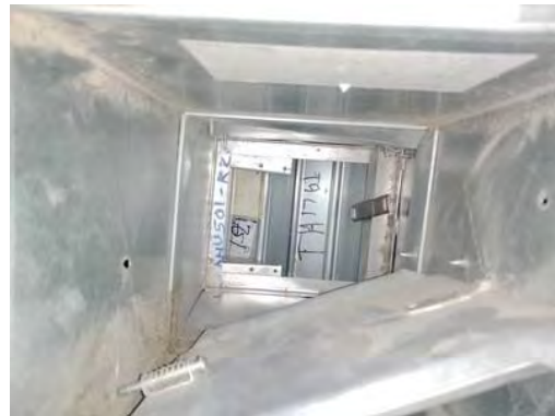
Picture of Damper I.D. Label
