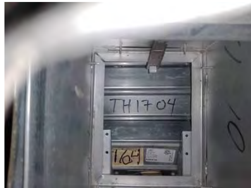
Picture of Damper I.D. Label
