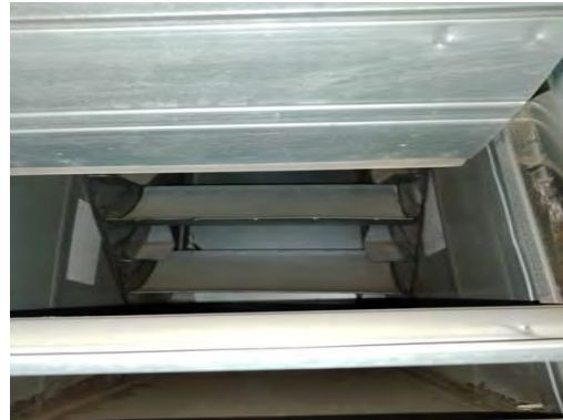
Picture of Damper in Closed Position
