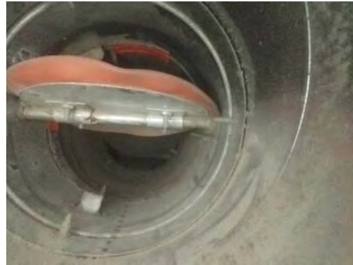
Picture of Damper in Closed Position
