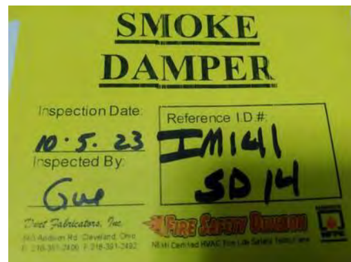
Picture of Damper I.D. Label
