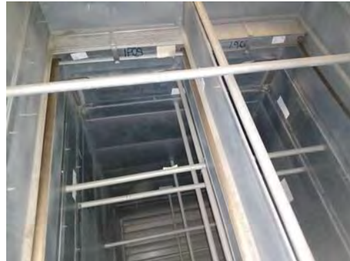
Picture of Damper in Closed Position
