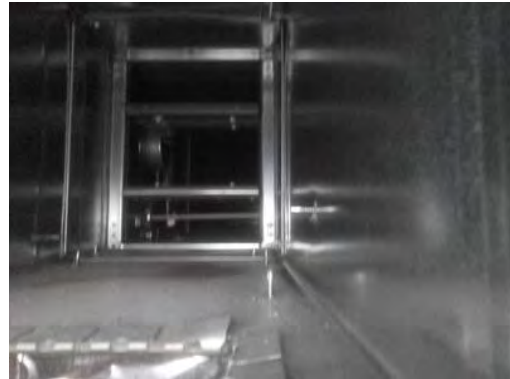
Picture of Damper in Closed Position
