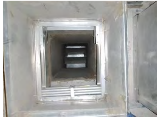
Picture of Damper in Closed Position
