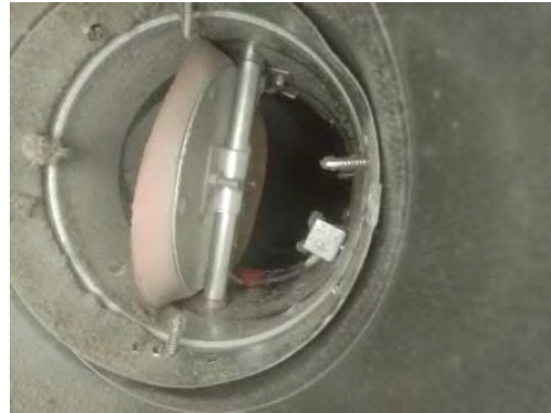
Picture of Damper in Closed Position
