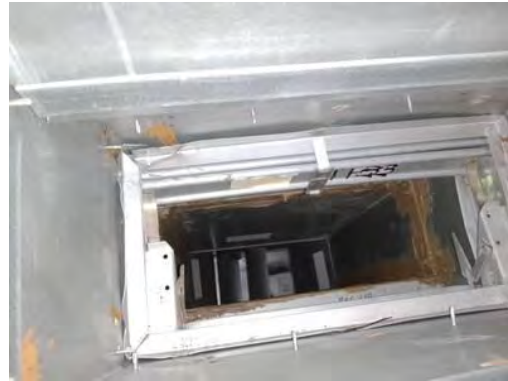
Picture of Damper in Closed Position
