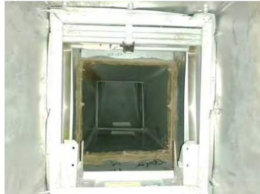
Picture of Damper in Closed Position
