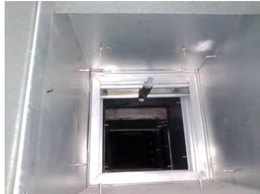
Picture of Damper in Closed Position
