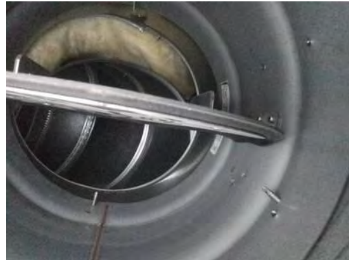
Picture of Damper in Closed Position
