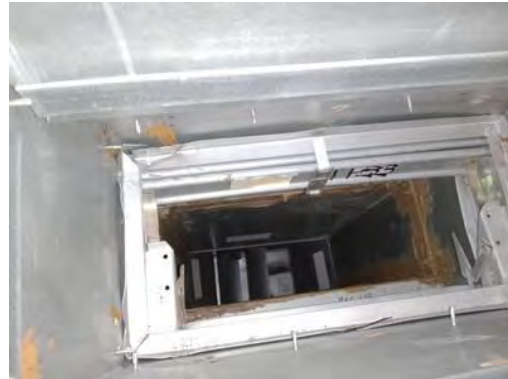
Picture of Damper in Closed Position
