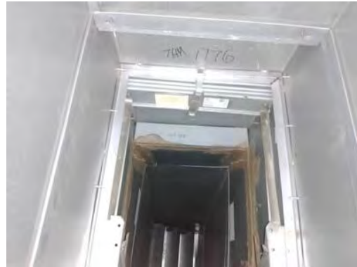
Picture of Damper in Closed Position
