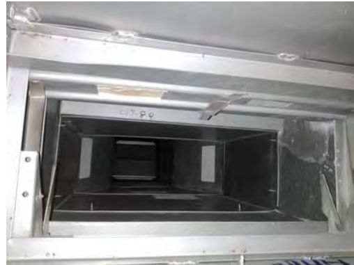
Picture of Damper in Closed Position
