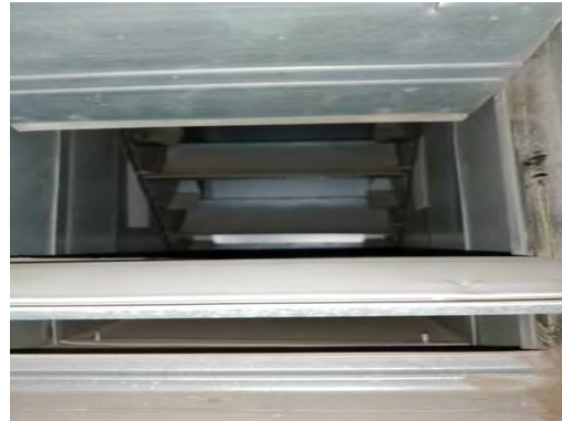
Picture of Damper in Closed Position
