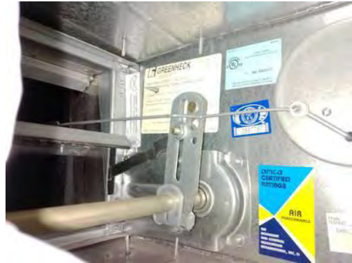
Picture of Damper in Closed Position
