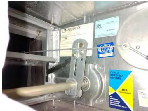
Picture of Damper in Closed Position
