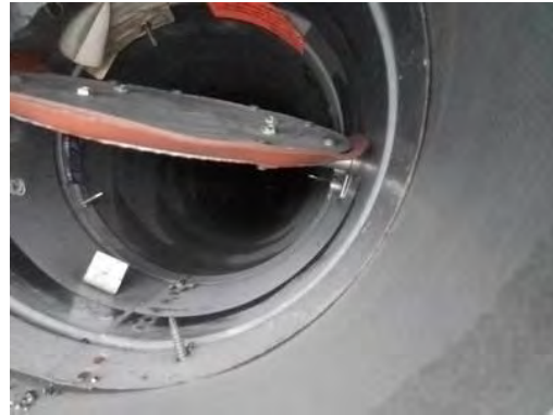
Picture of Damper in Closed Position
