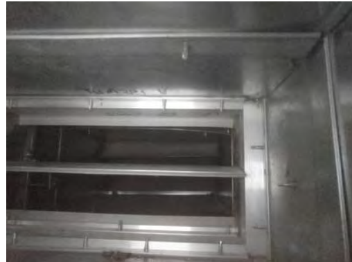
Picture of Damper in Closed Position
