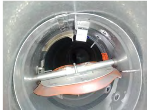
Picture of Damper in Closed Position
