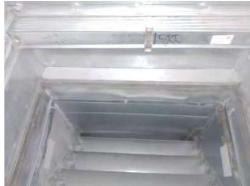
Picture of Damper in Closed Position
