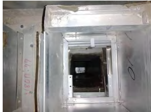
Picture of Damper in Closed Position
