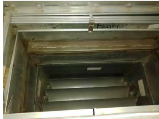
Picture of Damper in Closed Position
