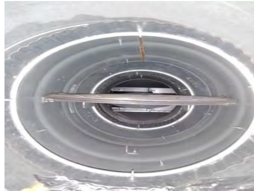
Picture of Damper in Closed Position
