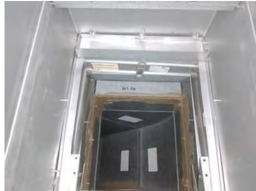
Picture of Damper in Closed Position
