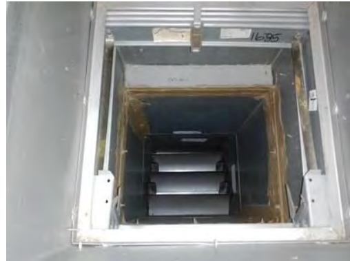
Picture of Damper in Closed Position
