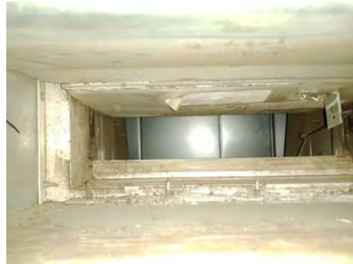
Picture of Damper in Closed Position
