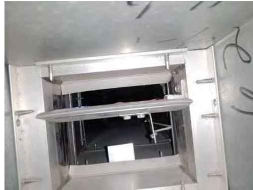
Picture of Damper in Closed Position
