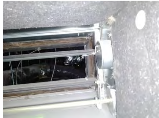
Picture of Damper in Closed Position
