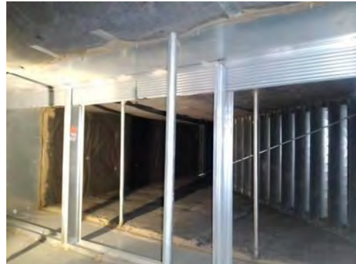
Picture of Damper in Closed Position
