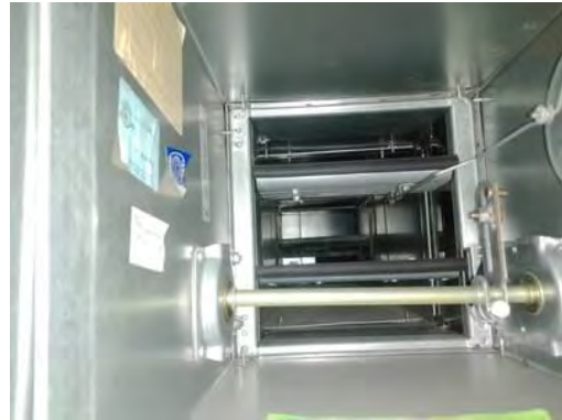
Picture of Damper in Closed Position
