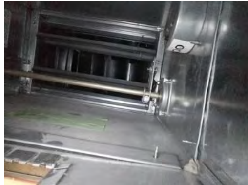
Picture of Damper in Closed Position
