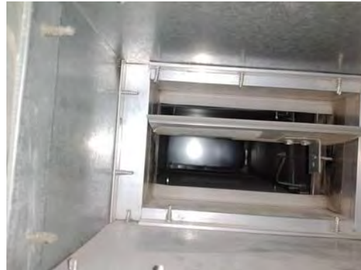
Picture of Damper in Closed Position
