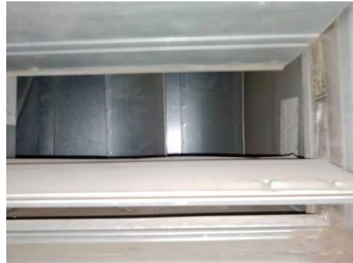
Picture of Damper in Closed Position
