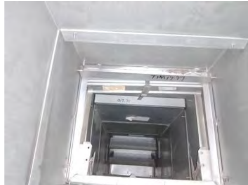
Picture of Damper in Closed Position
