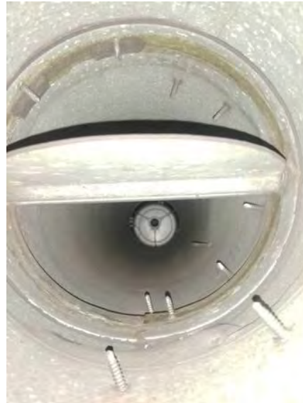
Interior Picture of Damper
