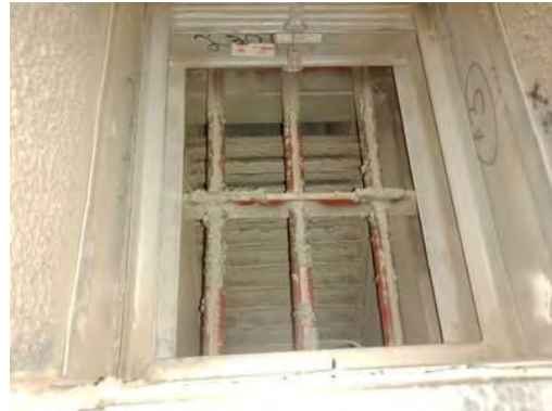
Interior Picture of Damper
