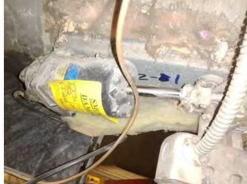
Interior Picture of Damper
