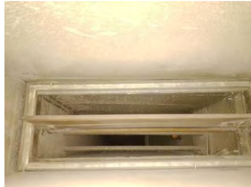
Interior Picture of Damper
