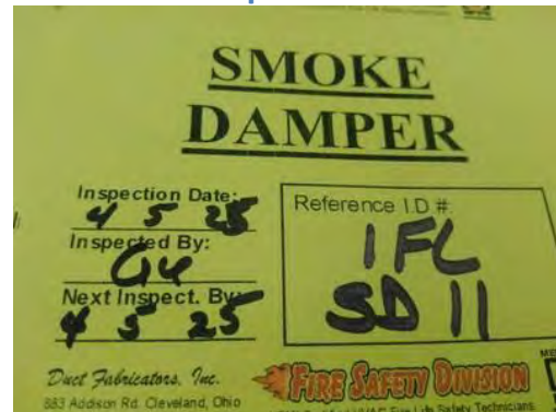
Picture of Damper I.D. Label
