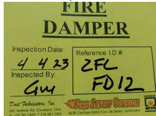
Picture of Damper I.D. Label
