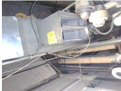
Interior Picture of Damper
