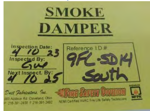
Picture of Damper I.D. Label
