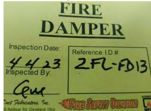
Picture of Damper I.D. Label
