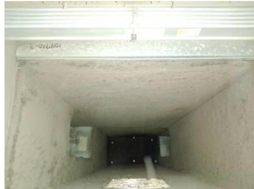
Picture of Damper in Closed Position
