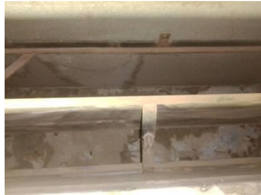
Picture of Damper in Closed Position
