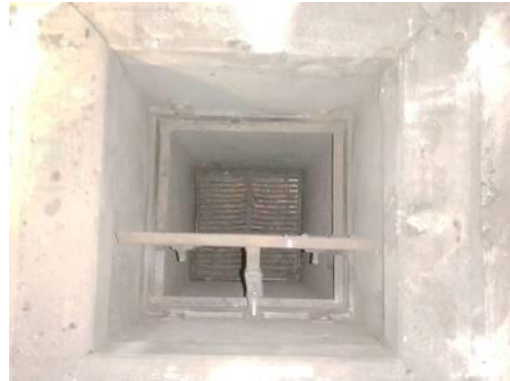
Picture of Damper in Closed Position
