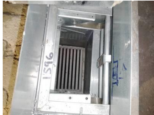
Picture of Damper in Closed Position
