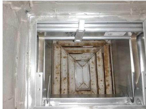
Picture of Damper in Closed Position
