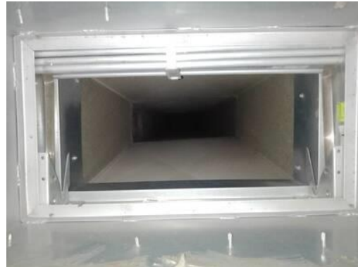
Picture of Damper in Closed Position
