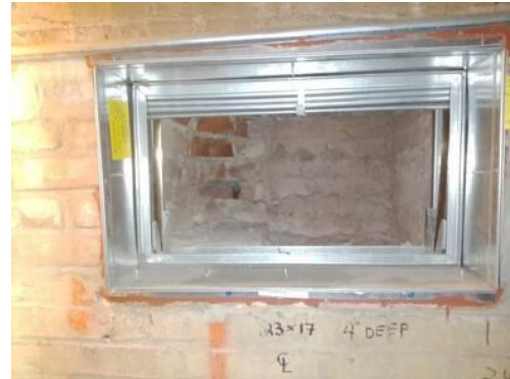
Picture of Damper in Closed Position
