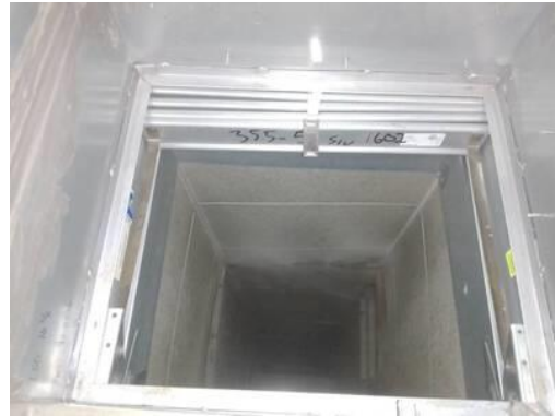
Picture of Damper in Closed Position
