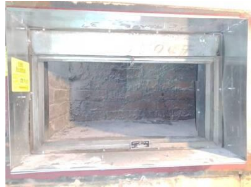
Picture of Damper in Closed Position
