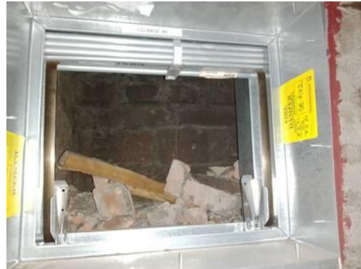
Picture of Damper in Closed Position
