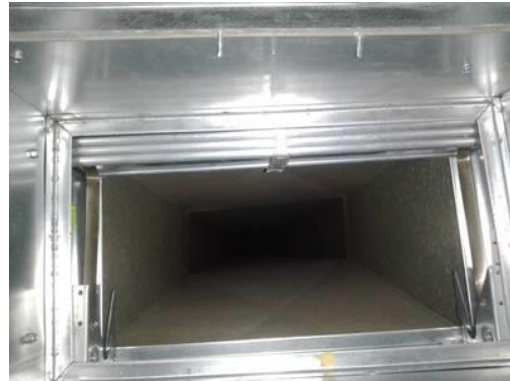
Picture of Damper in Closed Position
