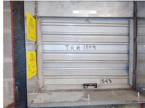
Picture of Damper in Closed Position
