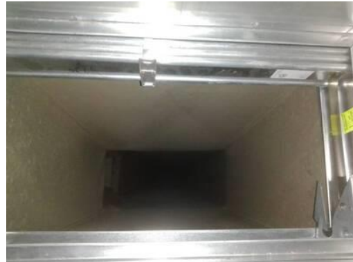
Picture of Damper in Closed Position
