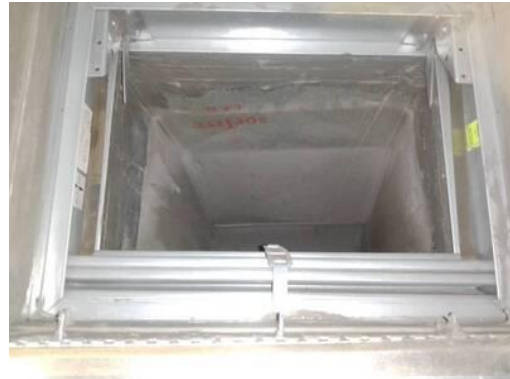
Picture of Damper in Closed Position
