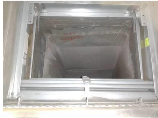
Picture of Damper in Closed Position
