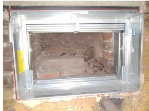
Picture of Damper in Closed Position
