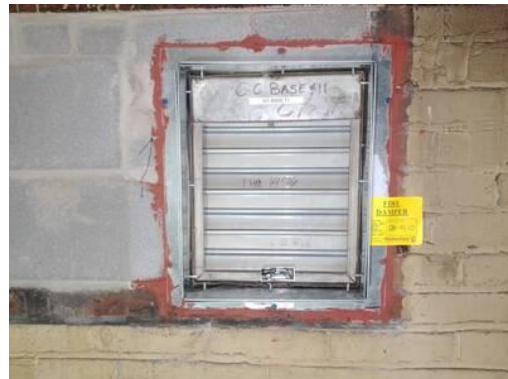
Picture of Damper I.D. Label
