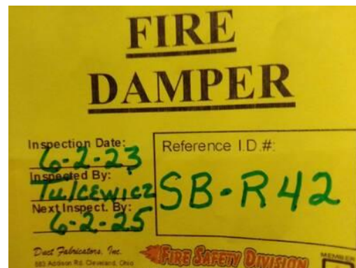
Picture of Damper I.D. Label
