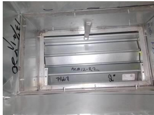
Picture of Damper I.D. Label
