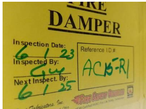
Picture of Damper I.D. Label
