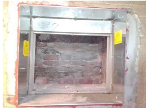
Picture of Damper in Closed Position
