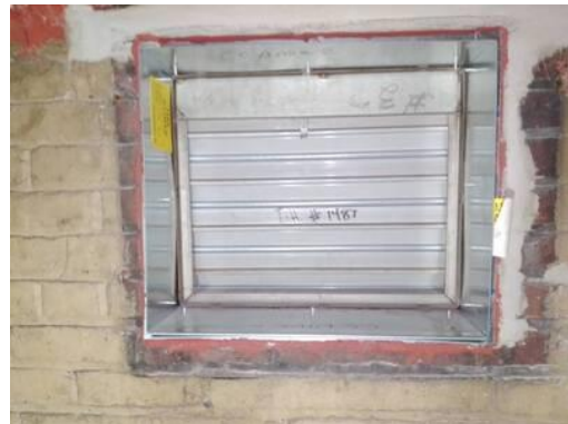
Picture of Damper I.D. Label
