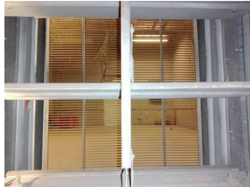
Picture of Damper in Closed Position
