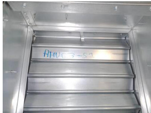
Picture of Damper I.D. Label
