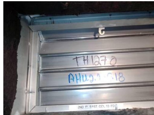
Picture of Damper I.D. Label
