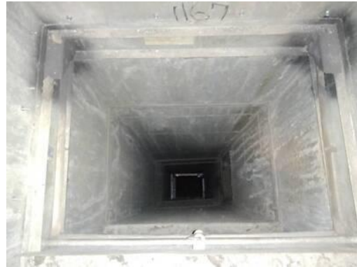
Picture of Damper in Closed Position
