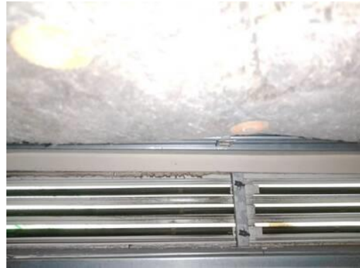
Picture of Damper in Closed Position
