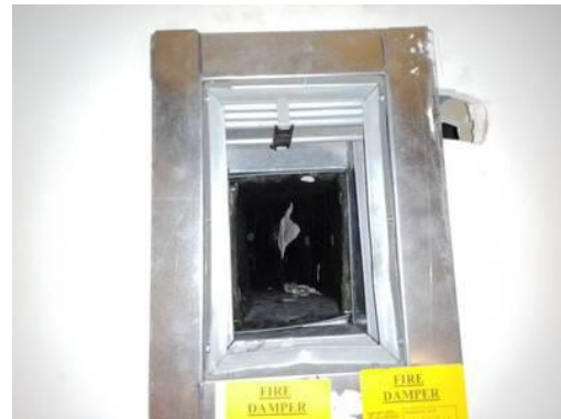
Picture of Damper in Closed Position
