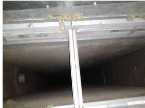
Picture of Damper in Closed Position
