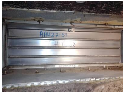
Picture of Damper I.D. Label
