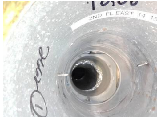
Picture of Damper in Closed Position
