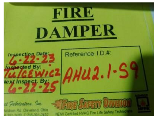
Picture of Damper I.D. Label
