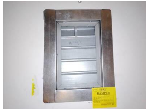
Picture of Damper I.D. Label
