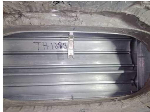
Picture of Damper I.D. Label
