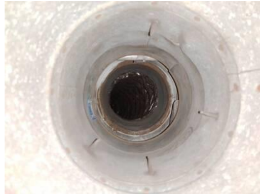
Picture of Damper in Closed Position
