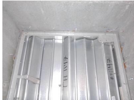
Picture of Damper I.D. Label
