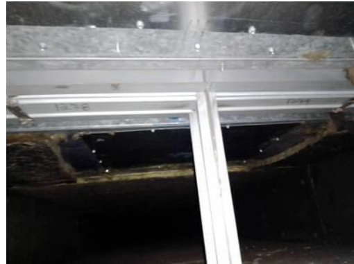
Picture of Damper in Closed Position
