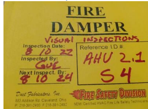
Picture of Damper I.D. Label
