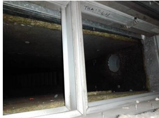
Picture of Damper in Closed Position
