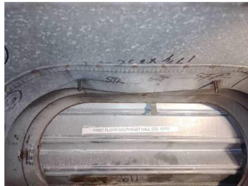
Picture of Damper I.D. Label
