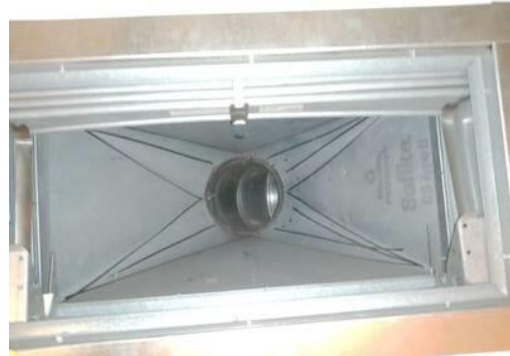
Picture of Damper in Closed Position
