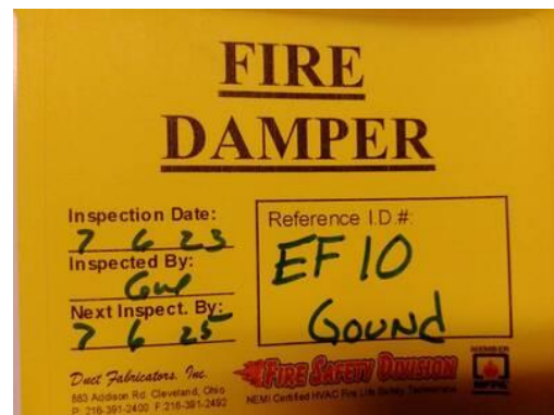
Picture of Damper I.D. Label
