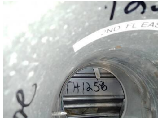
Picture of Damper I.D. Label
