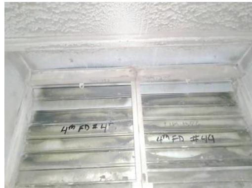
Picture of Damper I.D. Label
