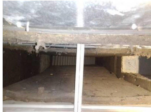
Picture of Damper in Closed Position
