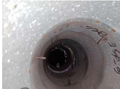
Picture of Damper in Closed Position
