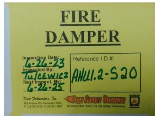
Picture of Damper I.D. Label
