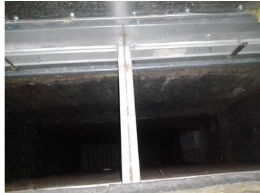
Picture of Damper in Closed Position
