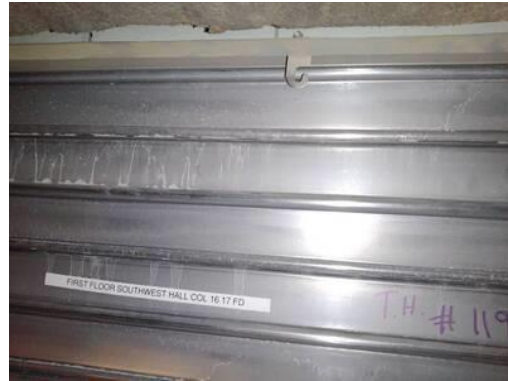
Picture of Damper I.D. Label
