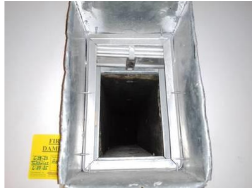
Picture of Damper in Closed Position
