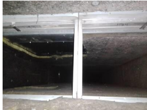
Picture of Damper in Closed Position
