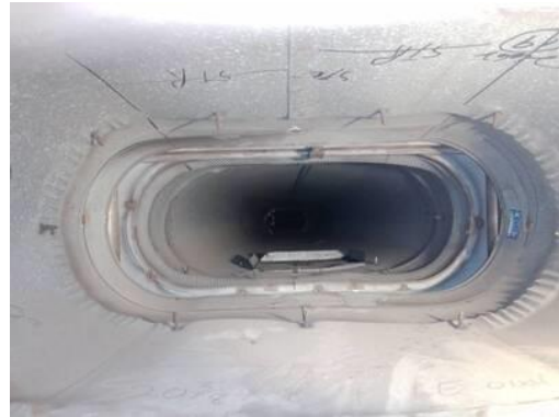
Picture of Damper in Closed Position
