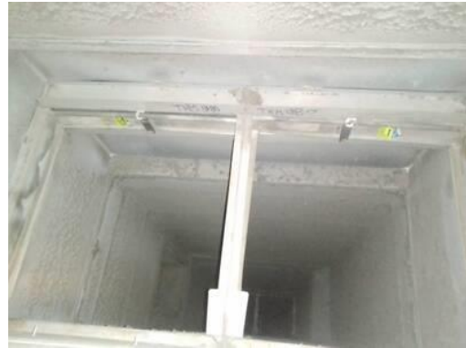
Picture of Damper in Closed Position
