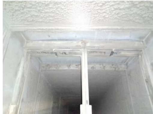
Picture of Damper in Closed Position
