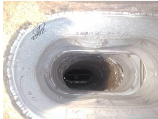
Picture of Damper in Closed Position
