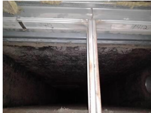
Picture of Damper in Closed Position
