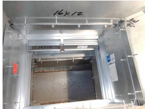
Picture of Damper in Closed Position
