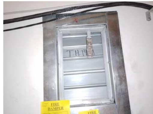
Picture of Damper I.D. Label
