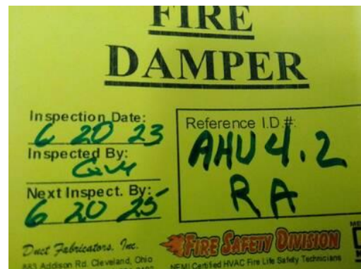
Picture of Damper I.D. Label
