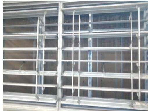
Picture of Damper in Closed Position
