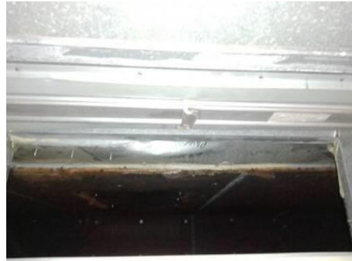
Picture of Damper in Closed Position
