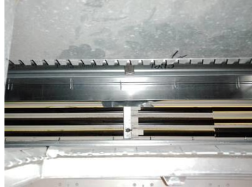
Interior Picture of Damper
