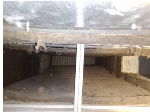
Picture of Damper in Closed Position
