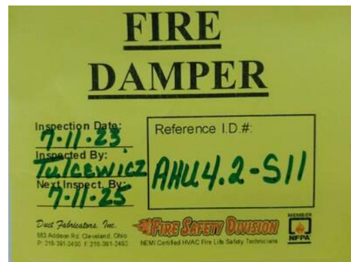
Picture of Damper I.D. Label
