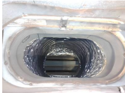
Picture of Damper in Closed Position
