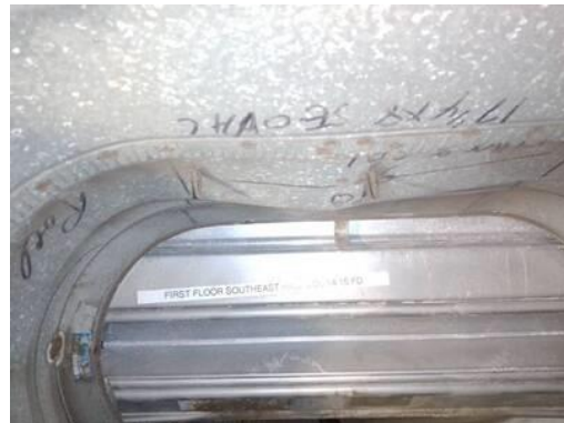
Picture of Damper I.D. Label
