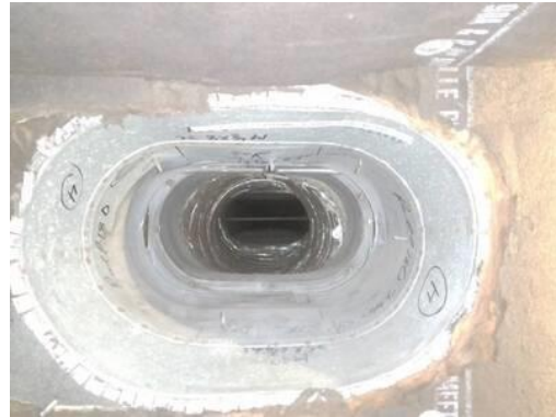
Picture of Damper in Closed Position
