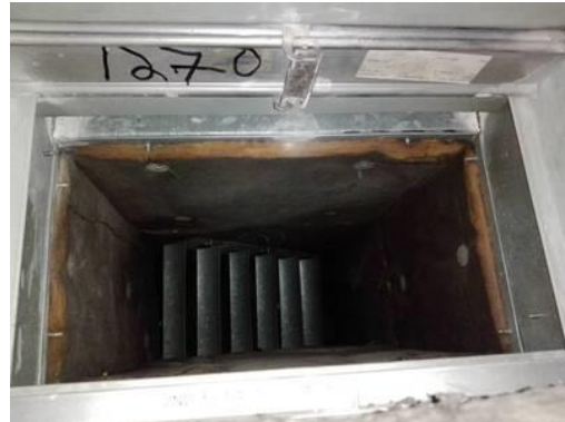
Interior Picture of Damper
