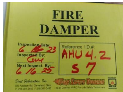
Picture of Damper I.D. Label
