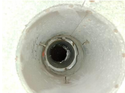
Picture of Damper in Closed Position
