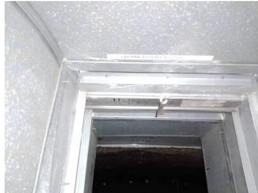
Picture of Damper in Closed Position
