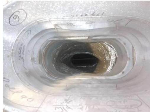
Picture of Damper in Closed Position
