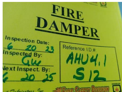
Picture of Damper I.D. Label
