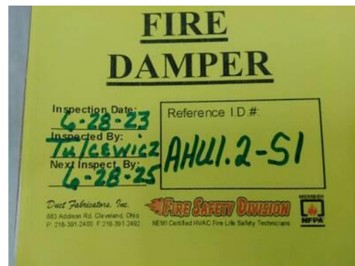
Picture of Damper I.D. Label
