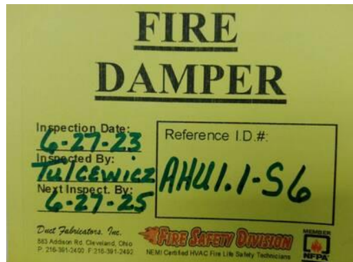
Picture of Damper I.D. Label
