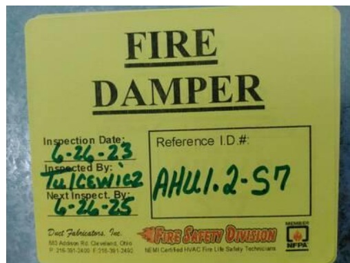
Picture of Damper I.D. Label
