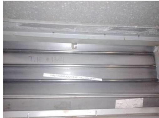
Picture of Damper I.D. Label
