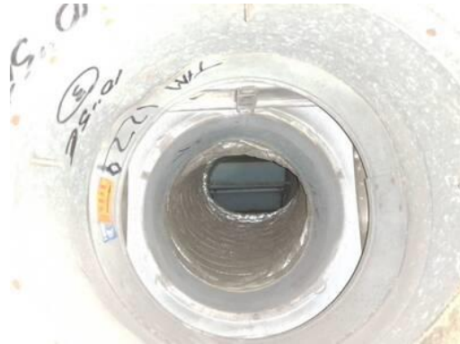
Picture of Damper in Closed Position
