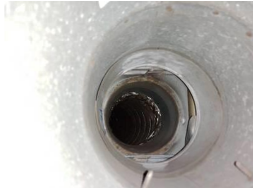
Picture of Damper in Closed Position
