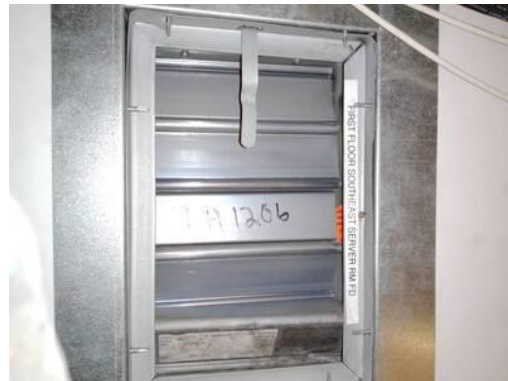
Picture of Damper I.D. Label
