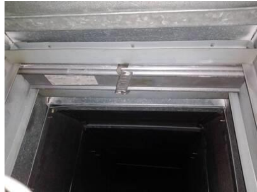
Picture of Damper in Closed Position
