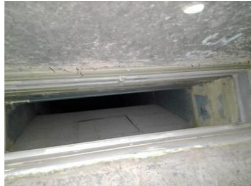
Picture of Damper in Closed Position
