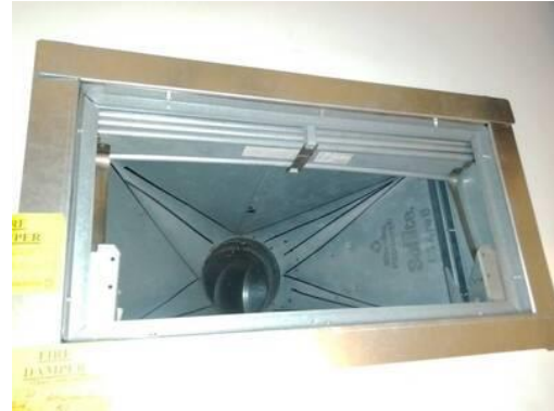
Interior Picture of Damper
