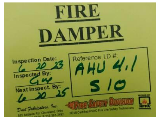
Picture of Damper I.D. Label
