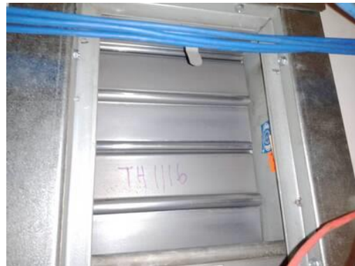
Picture of Damper I.D. Label
