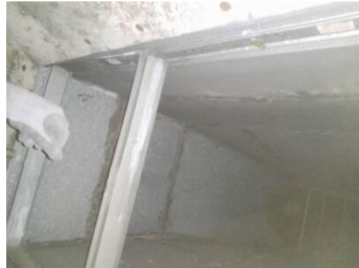
Picture of Damper in Closed Position
