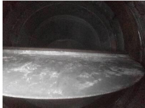
Picture of Damper in Closed Position
