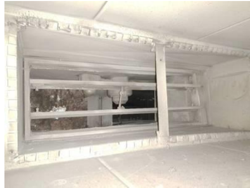
Picture of Damper in Closed Position
