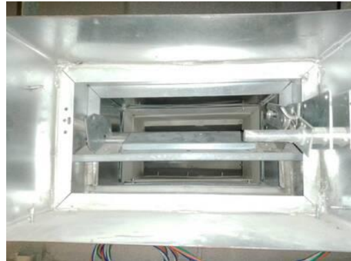
Picture of Damper in Closed Position
