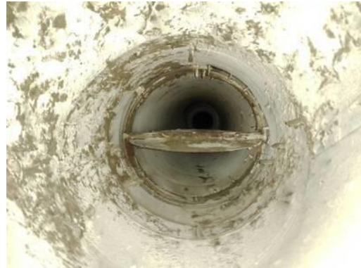
Picture of Damper in Closed Position
