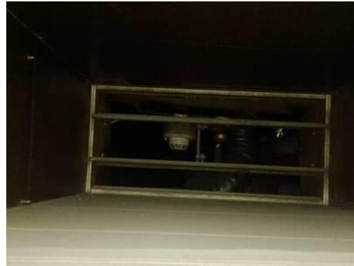
Picture of Damper in Closed Position
