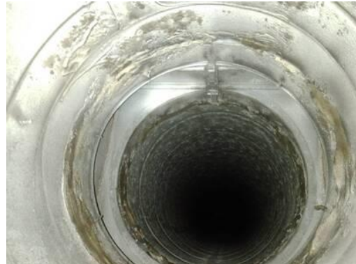
Picture of Damper in Closed Position
