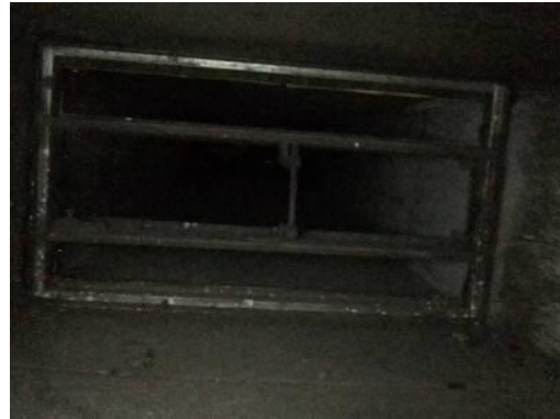
Picture of Damper in Closed Position
