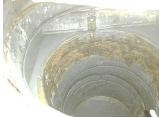
Picture of Damper in Closed Position
