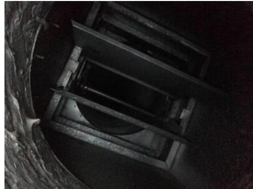
Picture of Damper in Closed Position
