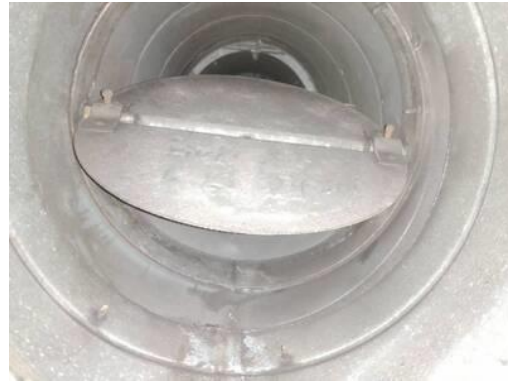
Picture of Damper in Closed Position
