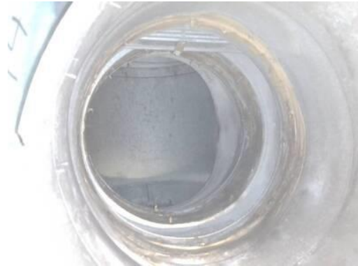
Picture of Damper in Closed Position
