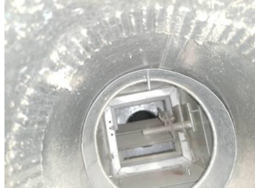
Picture of Damper in Closed Position
