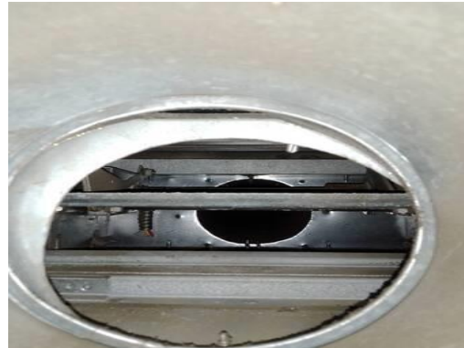
Picture of Damper in Closed Position
