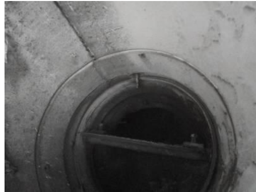
Picture of Damper in Closed Position
