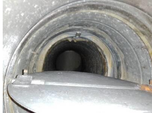
Picture of Damper in Closed Position
