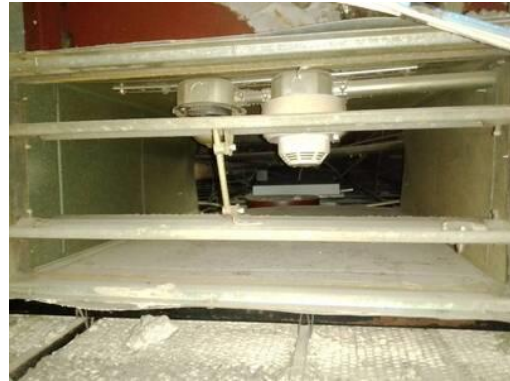
Picture of Damper in Closed Position
