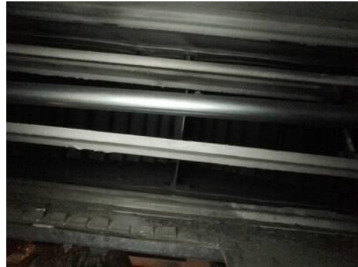
Picture of Damper in Closed Position
