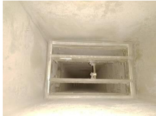
Picture of Damper in Closed Position
