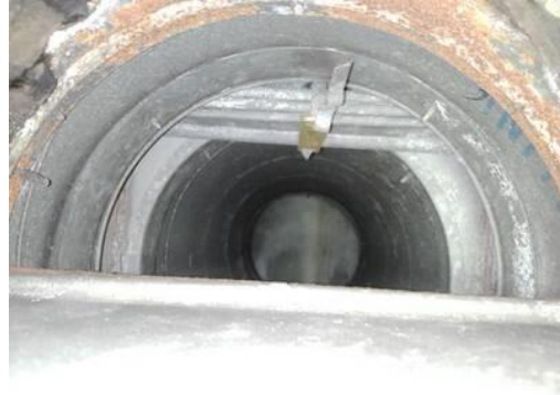
Picture of Damper in Closed Position
