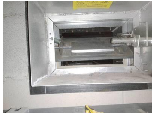
Picture of Damper in Closed Position
