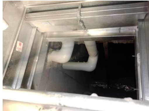
Picture of Damper in Closed Position
