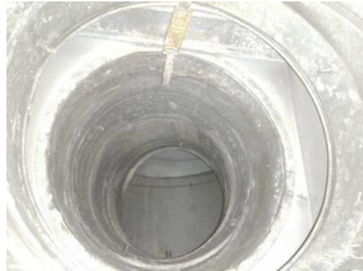
Picture of Damper in Closed Position
