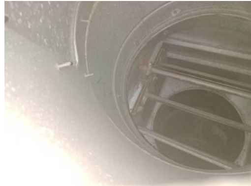
Picture of Damper in Closed Position
