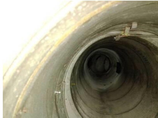
Picture of Damper in Closed Position
