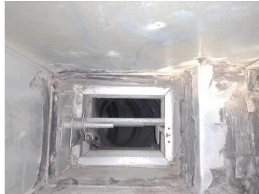
Picture of Damper in Closed Position
