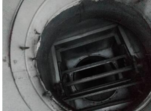
Picture of Damper in Closed Position
