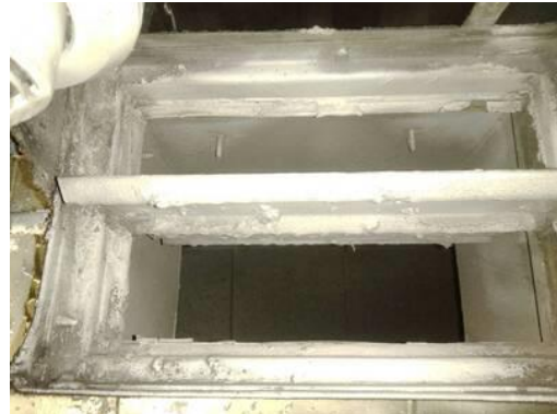
Picture of Damper in Closed Position
