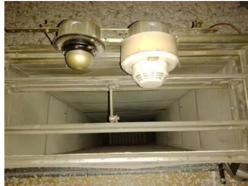
Picture of Damper in Closed Position
