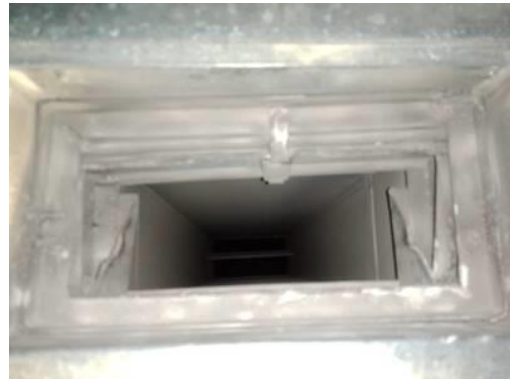
Picture of Damper in Closed Position
