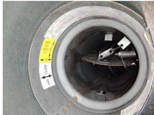
Picture of Damper in Closed Position
