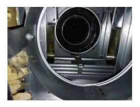
**Picture of Damper in Closed Position**
