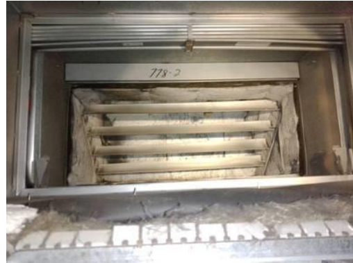
Picture of Damper in Closed Position
