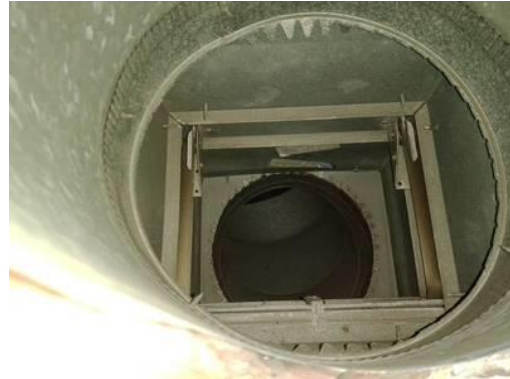
Picture of Damper in Closed Position
