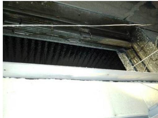
Picture of Damper in Closed Position
