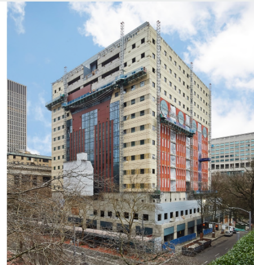
Utilized curtain wall installation 2019 (Sally Painter)
