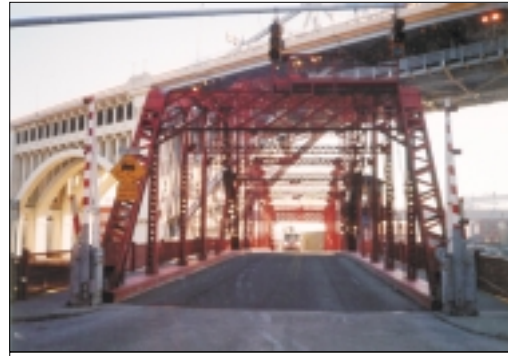
Center Street Bridge
