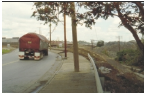
LTV entrance drive
