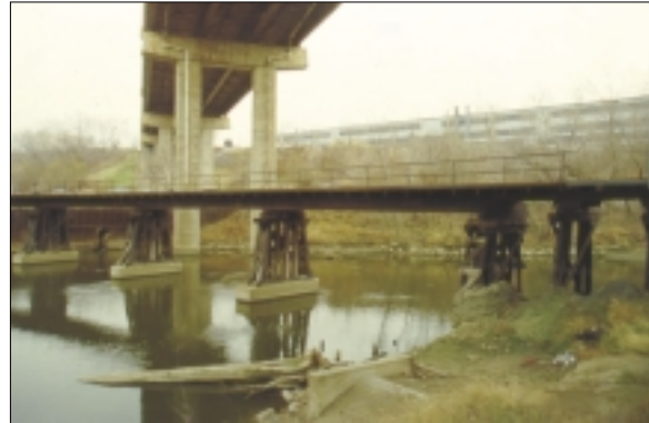
CSX Railroad bridge to clear near Harvard-Denison Bridge
