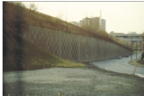
Interstate 71 retaining wall along LTV Drive
