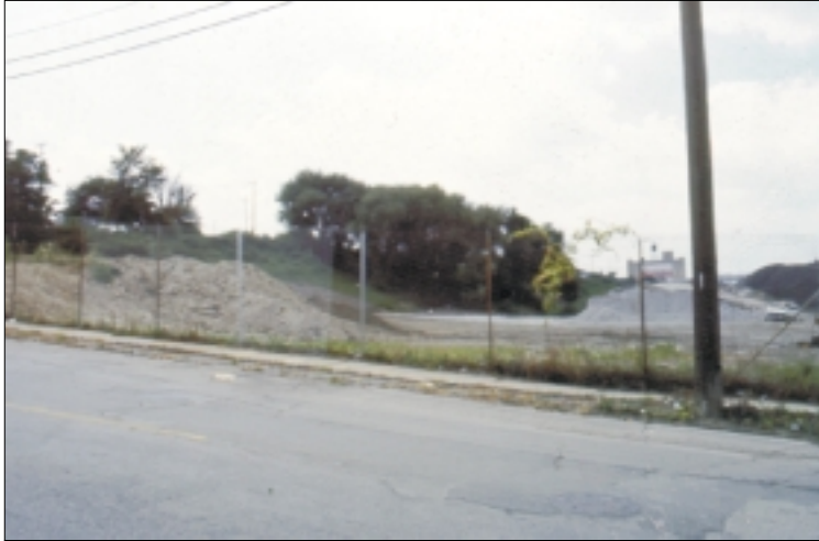
View from Literary Avenue into existing asphalt plant
