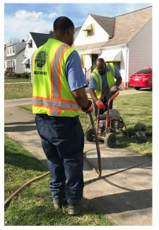
The Sewer Maintenance section provides a full-service program to clean, evaluate, maintain structural integrity, and perform construction on sanitary and storm sewers. The objective of the program is the cleaning of all sanitary sewers every three years and performing video inspection every six years which is well within the NEORSD's *"Best Management Practices"* guidelines.
