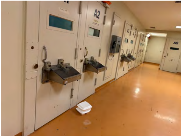
Jail I, Housing Unit 10A2 with secure food traps and cell door signage
