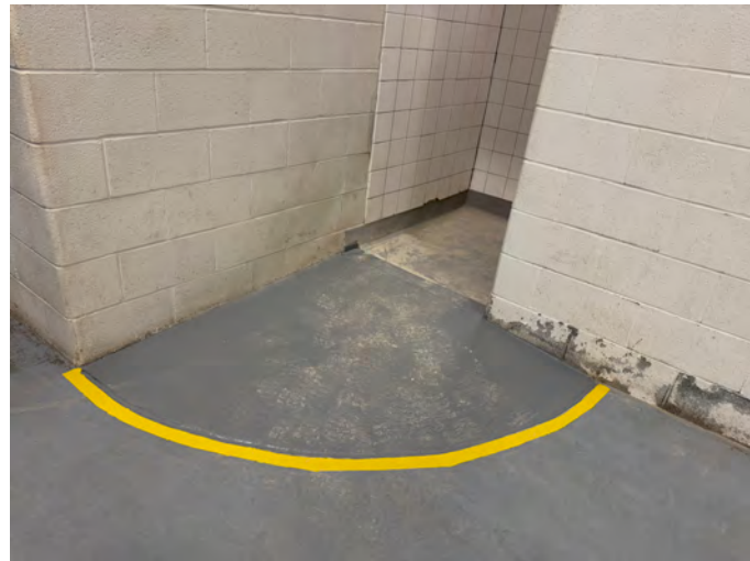
Renovated shower with wheelchair accessible ramp.
