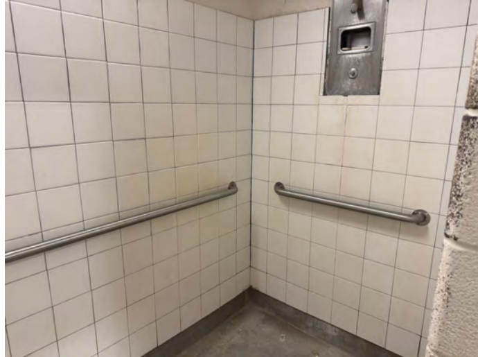
Renovated shower with grab bars.
