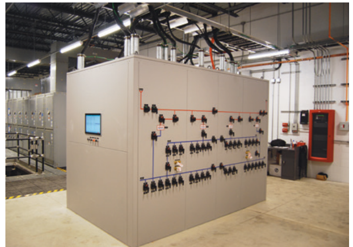
Duplex control board complete with HMI, control switches and 69kV relays (on opposite side, not shown)
