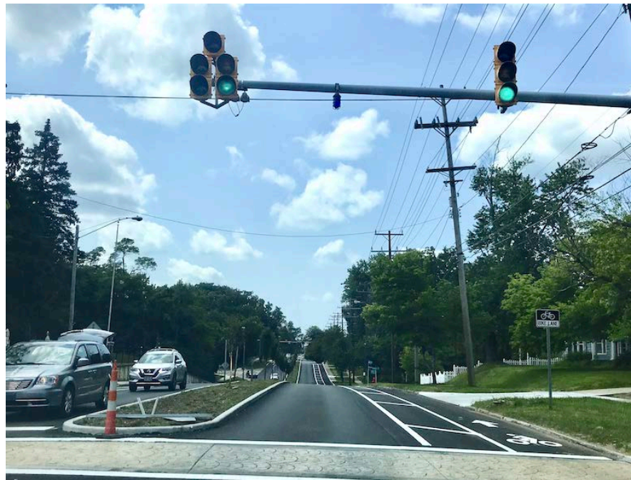
A 'road diet' in Parma Heights led to a planted median and bike lanes
