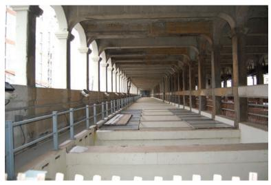
CANTILEVERED SECTIONS OF THE BRIDGE have an open decking system that would need to be fenced off or partially covered to prevent people from gaining access or falling through.
