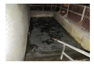
MOISTURE LEVELS, due to flooding, have effected the concrete structure and subsequently the re-bar, particularly in the western embankment
