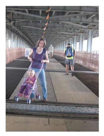
PLYWOOD SURFACE over the grated deck at the center span is difficult to navigate with bicycles, wheelchairs, and strollers. A continuous, non-skid surface needs to be installed to provide full accessibility across the bridge.
