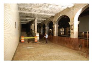
WITH A RAMP SLOPE OF 16%, the approach for cyclists to merge into the bridge would be unsafe, given column spacing and the landing area at the base of the ramp
