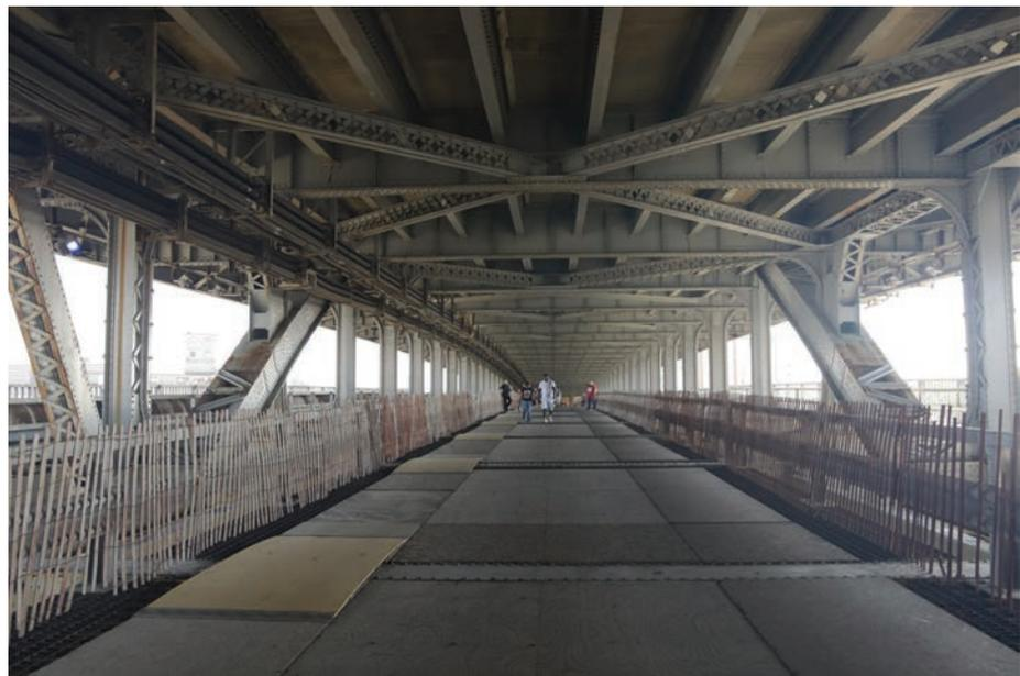
Ramps over the gaps between plywood sheets along the southern edge of the center span.
